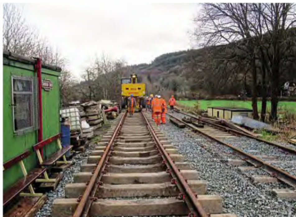
Double track now in place on the approach to Corwen. GEORGE JONES
