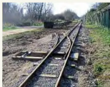
The lower station of the Royal Arsenal Narrow Gauge Railway now under construction. RANG
