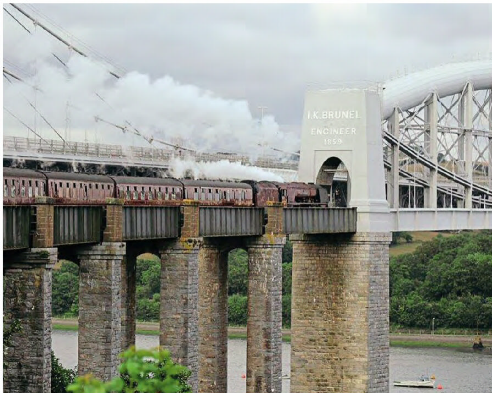
Princess Coronation Pacific No. 6233 Duchess of Sutherland slowly makes its way on to the Royal Albert Bridge with the 'Royal Duchy' on July 21. HENRY HOWE
