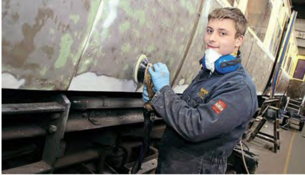
George Brogan, who has completed his four-year apprenticeship this summer, takes a break from sanding GWR inspection saloon No. 80869 inside the paintshop at Kidderminster and poses for the camera. GARETH EVANS
