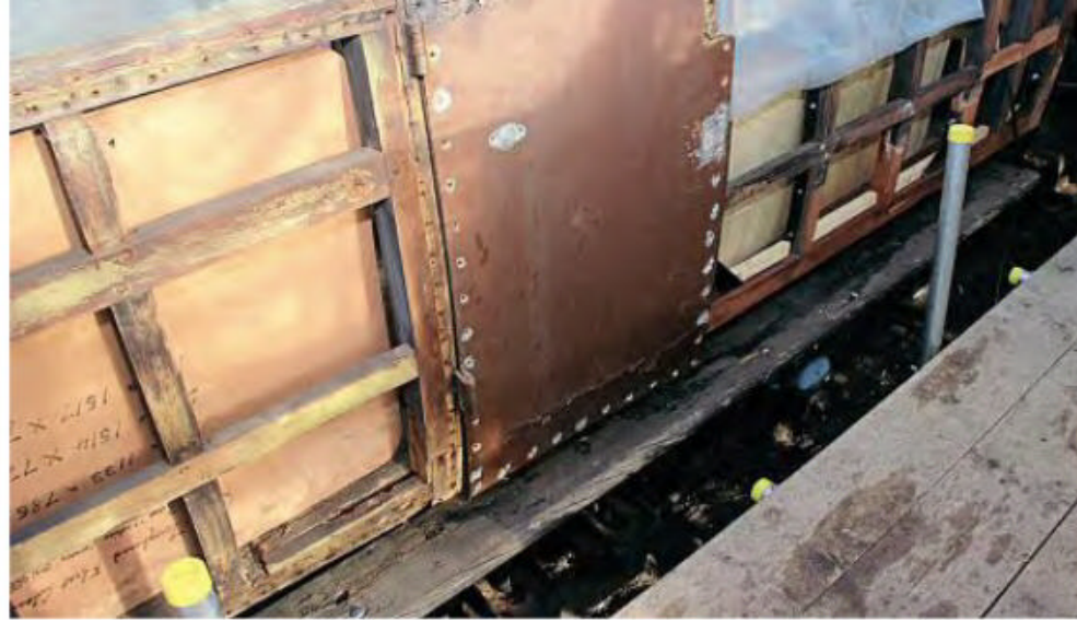
The restoration of 1926-built GWR Collett bow-ended Third No. 4786 at Bewdley has involved attending to corrosion at the bottom of the bodysides – the result of bolts and brackets rusting. GARETH EVANS
