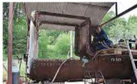
The outer wrapper of the firebox of No. 563 being removed at the Flour Mill workshop. BILL PARKER
