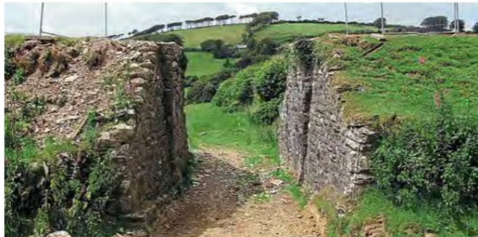
The initial work undertaken by the railway's 'Thursday gang' to expose the original foundations to the Lynton abutment of Bridge 54 was completed with the aid of a 32-tonne excavator. L&B
