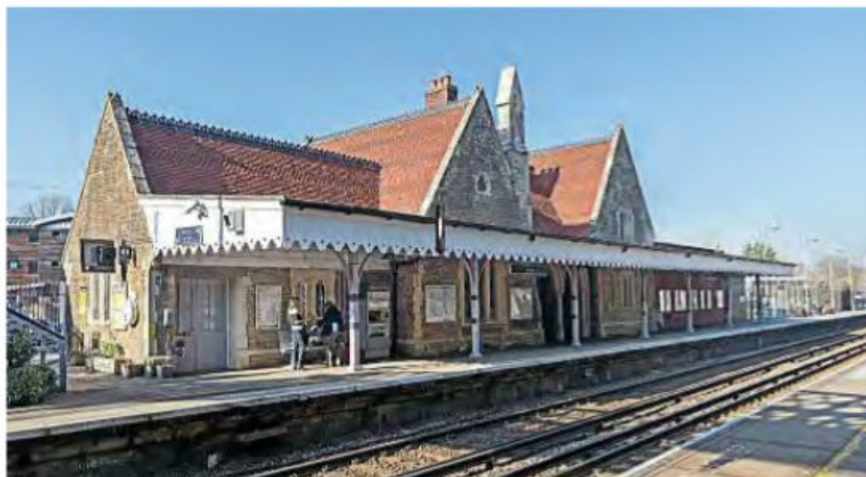
Battle stations: It may be 167 years old, but Grade II-listed Battle station in East Sussex looks as good as new after a major conservation project described by local MP Huw Merriman as "remarkable".
