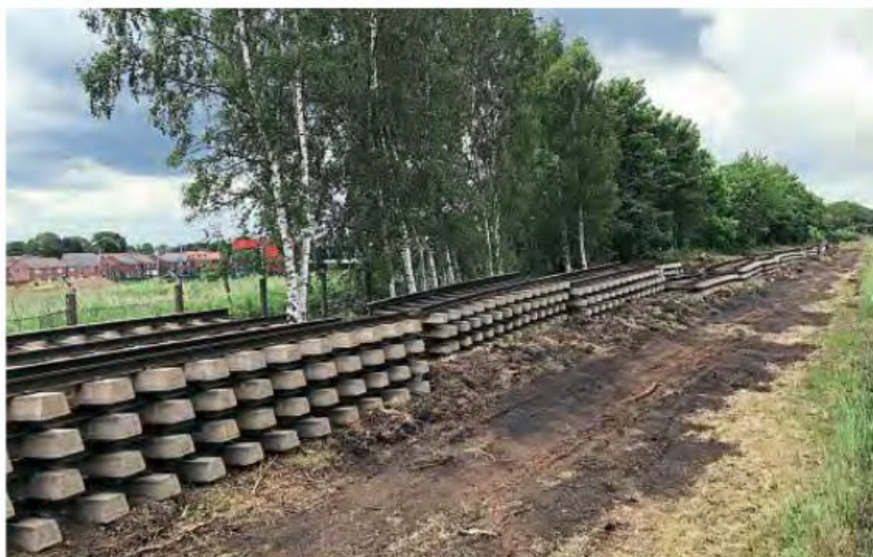
The track panels from Network Rail, stored alongside the SVR's formation at the site of the old sugar beet factory. PAUL APPLETON
