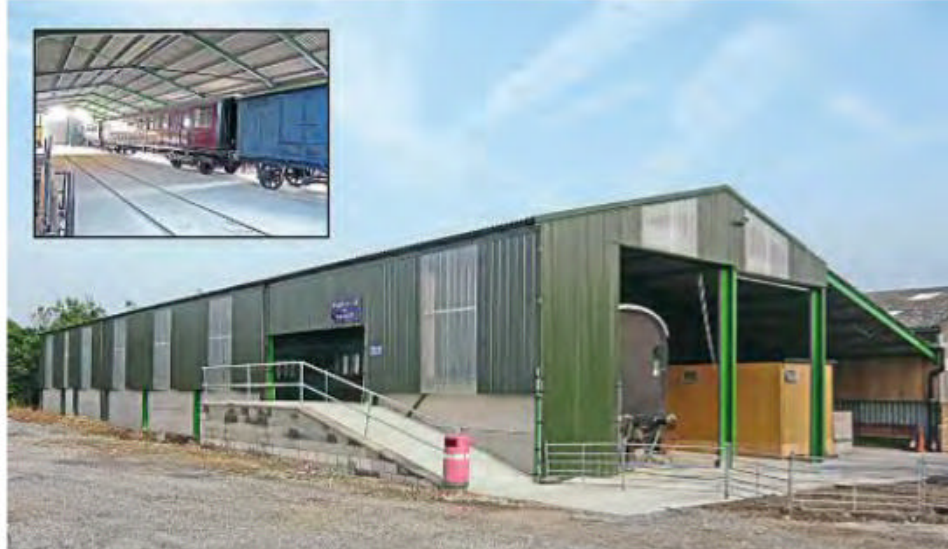
Space for more: The three-road carriage shed being built at Mangapps Railway Museum in Essex as part of a major expansion programme. Inset: The interior of the shed, which is already in partial use. Nearest the camera is an ex-Norwich Eastern Railway perishables van, built about 1900, that in 1943 was converted into a rectifier van and later a stores van, in which guise it sat in a siding at Norwich Thorpe for more than four decades before being acquired by John Jolly. Behind this veteran is a 1929 LNER Gresley teak coach, and then a 1921 LSWR brake third. JOHN JOLLY
