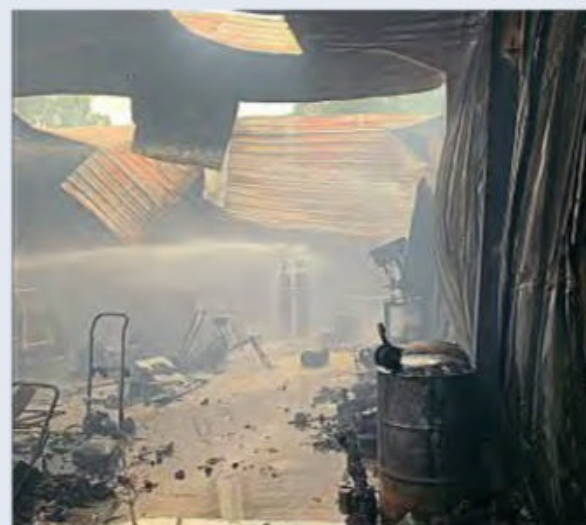
The damaged Boat of Garten workshop. ANDREW DICK/SCOTTISH FIRE & RESCUE SERVICE
