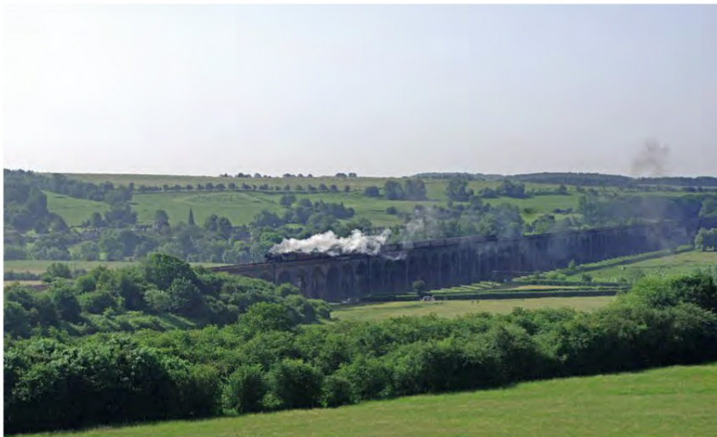
National Collection-owned A3 Pacific No. 60103 Flying Scotsman crosses Harringworth Viaduct, also known as Welland or Seaton Viaduct, on June 29. ROBIN JONES
