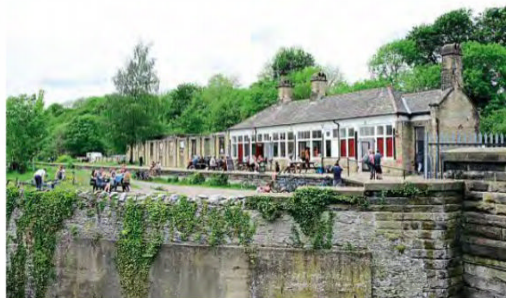
The ticket office at Millers Dale station on the Monsal Trail in Derbyshire which has become a popular cafe. BRIAN SHARPE
