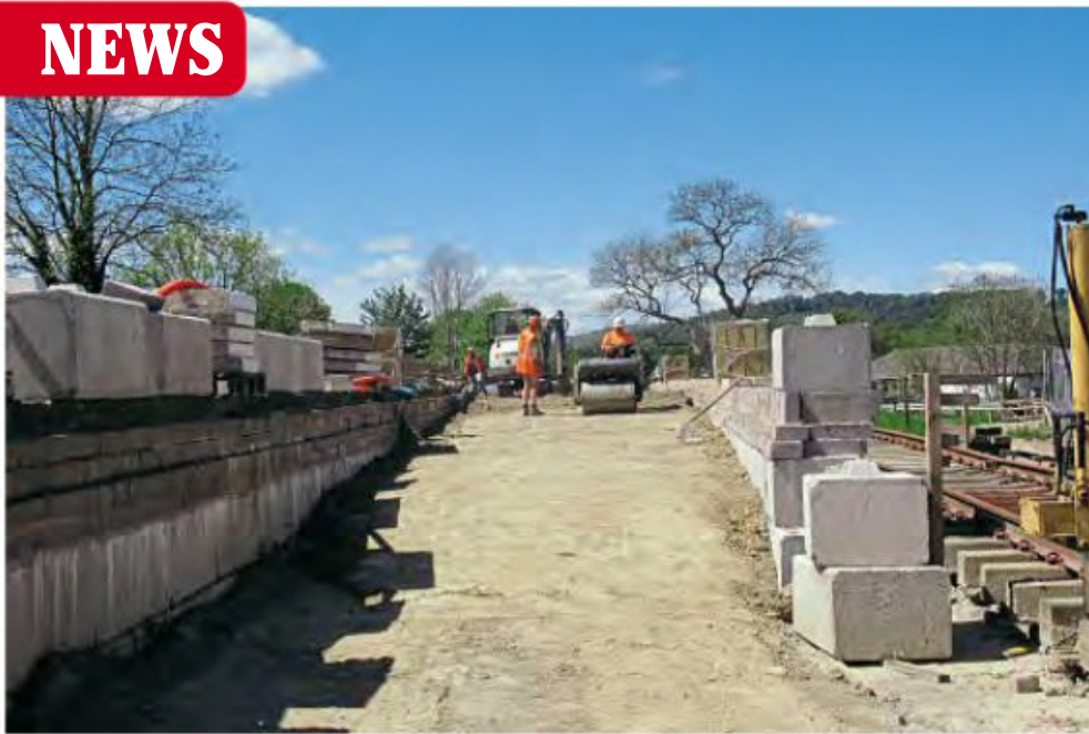
Gap no more: the formation of the Llangollen Railway can now lead straight into Corwen Central station, with platform construction seen taking place. LR
