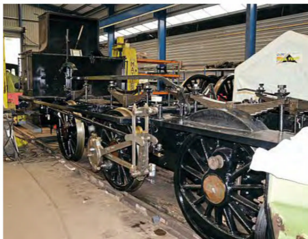
No. 656 is seen inside Wansford works with the bunker and valve gear in place. NATHAN WILSON/NVR
