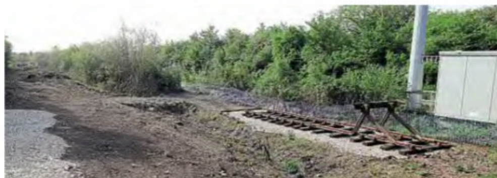
Statement of intent: Aylesbury & Buckingham Railway trackbed clearance, a buffer stop and a token track panel marks the first stage of a planned northern extension for the Buckinghamshire Railway Centre's running line. LENNY BARKER
