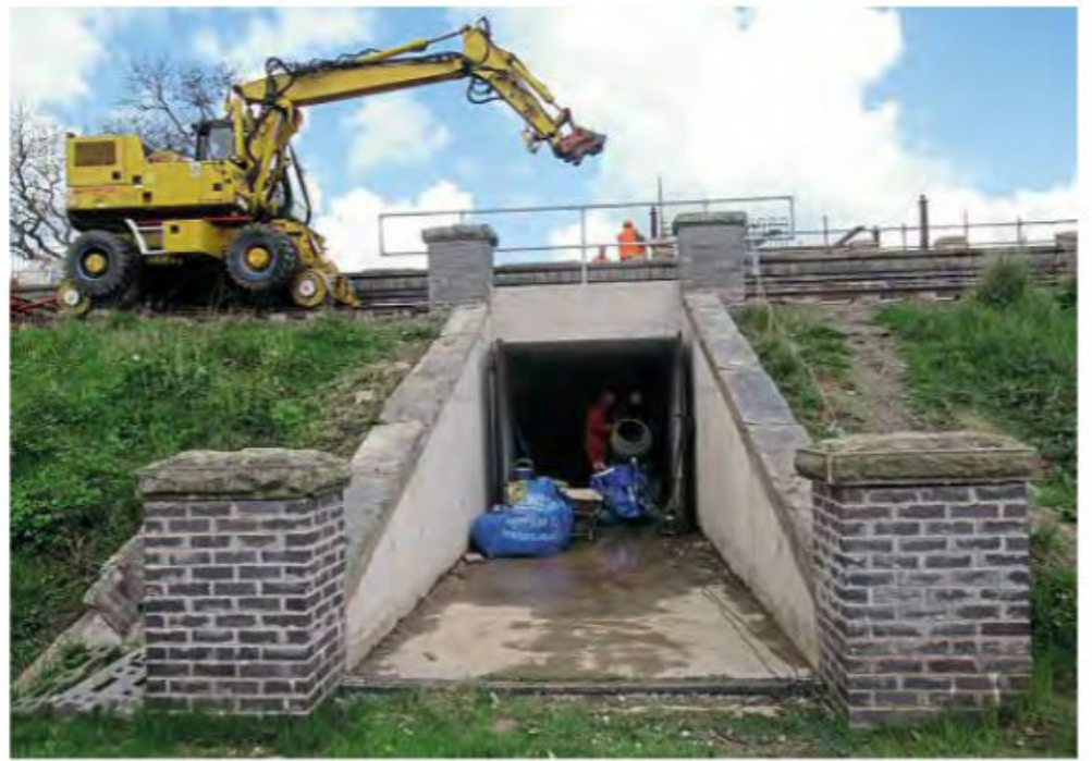
The underpass at the new Corwen Central station. LR
