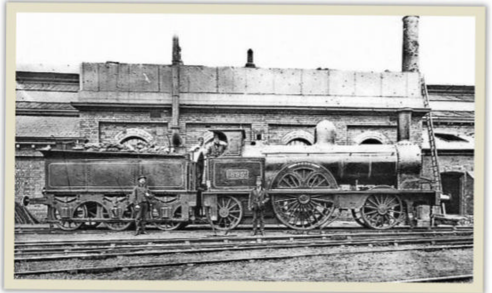
Large Bloomer No. 895 Torch at Birmingham's Monument Lane shed in 1877.
