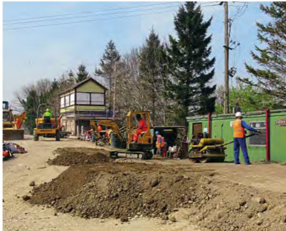
Looking west over the gap, showing the depth of the infill to level up.
