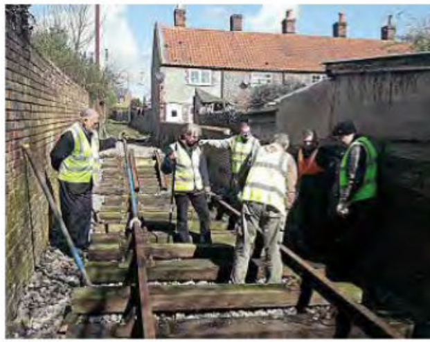
Volunteers working on the first length of the reborn Leiston Works Railway. LWR
