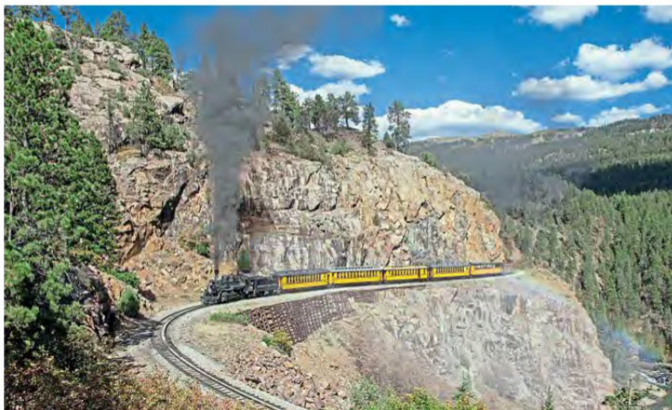
The most dramatic part of the Cumbres & Toltec is 'The High Line' just north of Rockwood, which runs on a ledge 400ft above the Animas River. This section of track was the most expensive to build – there being a need to blast through the hard red rock to create the shelf cut into the steep cliff face over the river. No. 476, built by Alco in 1923 works along 'The High Line' on September 23.
