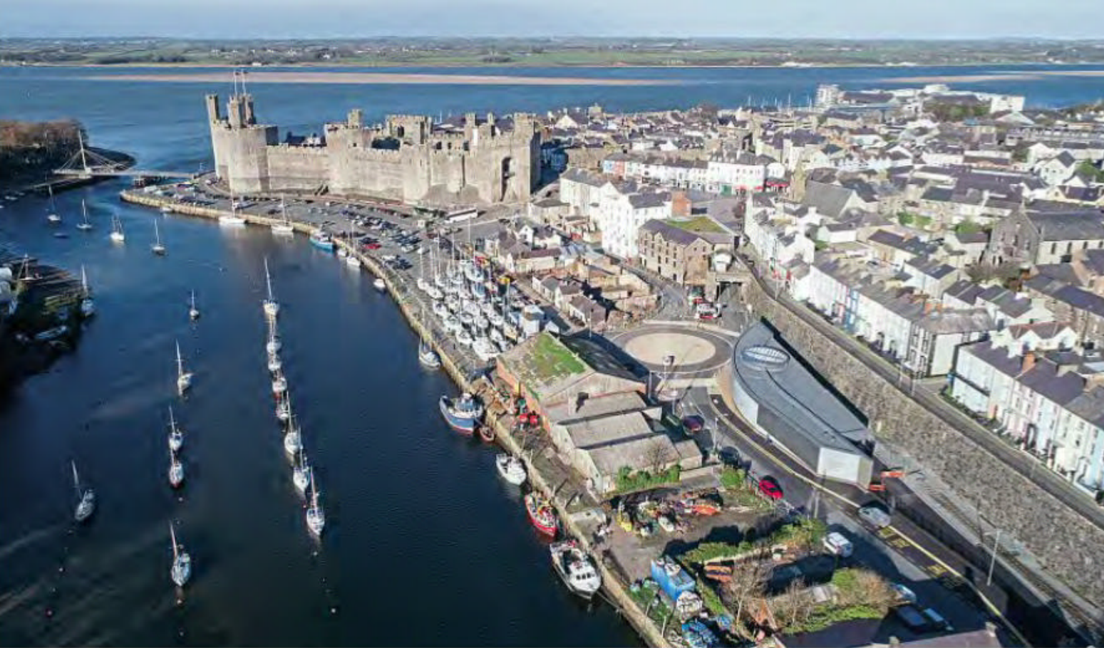
An aerial view highlighting the position of the new Welsh Highland Railway terminus in Caernarfon. FF&WHR
