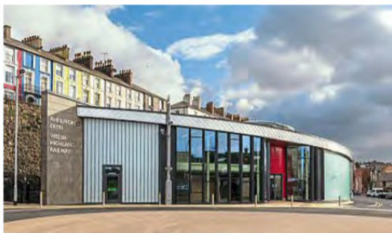
A 21st-century terminus for the modern-day Welsh Highland Railway. FF&WHR
