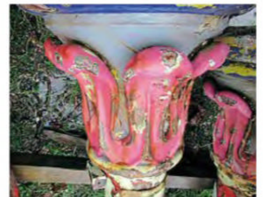
The restored Acanthus decoration on the top of the columns from Blackfriars station. LR
