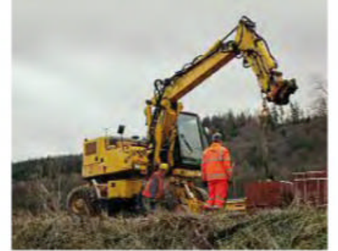
A Rexquote Superailer road-rail crane/excavator is now active on the Corwen station site and has traversed both sides of the platform via the Green Lane headhunt. It has been brought in for use within the existing rail loop as the means to deliver materials along the platform area now that the road vehicles are restricted within the development. Its first use was at the west end of the loop preparing to lift pallets of pavers which will be laid to provide the final surface of the island platform. GEORGE JONES/LR
