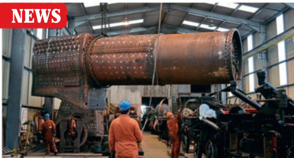
After more than 18 months' work at Tyseley Locomotive Works, the overhaul of the boiler from No. 7927 Willington Hall is lowered into the frames of No. 6880 Betton Grange for trial fitting on December 3. LYNN MOORE
