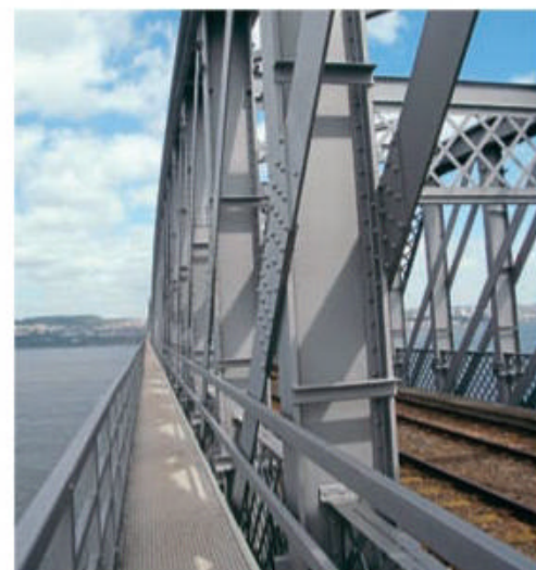
A view of the new walkway and the high girders on the Tay Bridge at Dundee which won the top prize, this year in honour of the late Sir William McAlpine. NRHA
