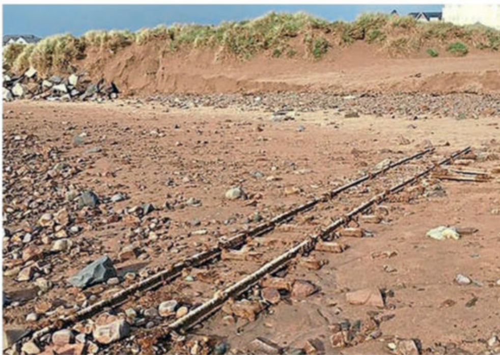
One of the narrow gauge track panels exposed on Summerleaze Beach at Bude. NICKY COOTE
