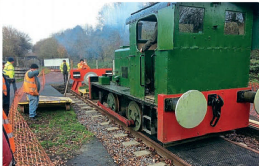
Two days after the panels were installed, the railway's Fowler 60hp diesel shunter Progress (No. 4000001 of 1945) made the first run over the new crossing. TVR
