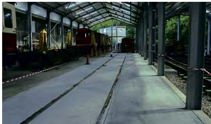
The first two roads in the new shed are tramway laid maintenance roads for bogie overhauls and the like – work which was previously undertaken outdoors. COLIN TYSON
