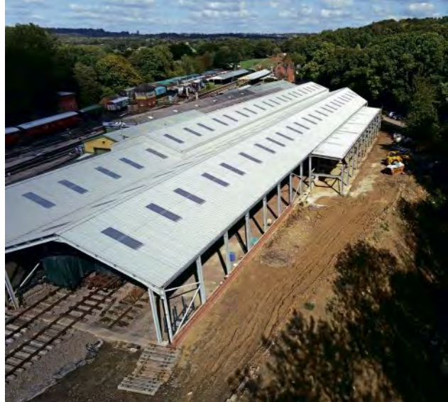
RIGHT: The new carriage shed at Horsted Keynes, showing the made-up ground to the right to provide an access road, now awaiting the pointwork to provide the last two roads into the shed. BRT
