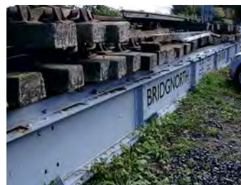
The former Bristol (Bath Road) turntable has been released from the undergrowth at Eardington station and been given a superficial coat of fresh paint to tidy it up. It is planned to overhaul the turntable and install it into a newly-constructed pit in the shed yard at Bridgnorth.
