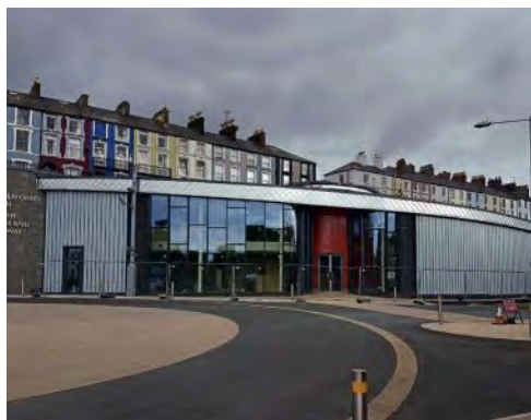
The striking modern design of the new Caernarfon station building. The need to keep the station height below a level so as not to impact on the view from the cottages above is apparent in this view, taken on September 30. The coach bay is located out of shot to the right. PAUL LEWIN
