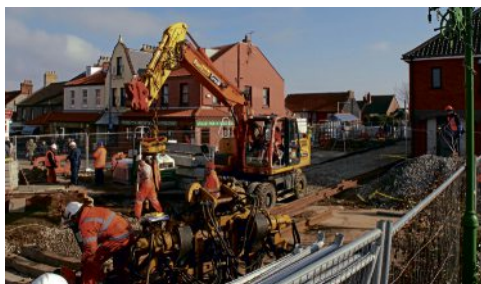
Above: Work is progressing well on reinstating the missing link and level crossing at Sheringham in February 2010.
