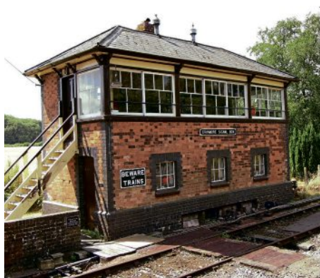
The charming GWR Cranmore signal box, which is at one end of the new platform that's being built.
