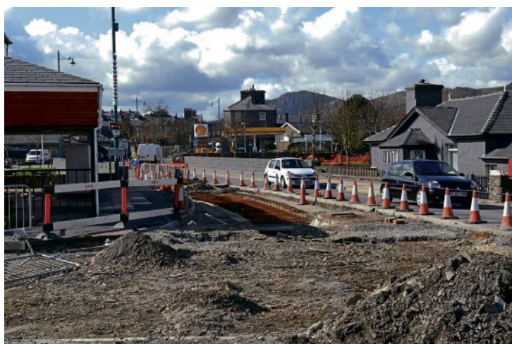
By 2008 the route of the reinstated Welsh Highland Railway through Porthmadog was becoming clearer and the first section of track is about to be laid across the Britannia Bridge on the approach to Harbour station.
