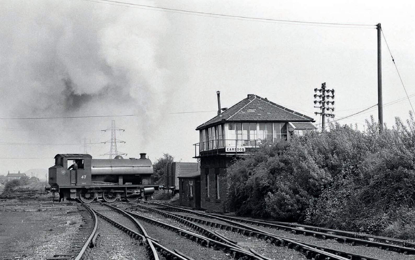
NCB Robert Stephenson & Hawthorns-built 0-6-0ST (No. 7849 of 1955) No. 47 crosses over the Blyth and Tyne at Earsdon with a train from Fenwick Colliery on August 28, 1970. Built for the Northumberland Area of the National Coal Board, it was originally used at Backworth Colliery, near Whitley Bay, where it had a royal blue livery and carried the number 47. It later moved to Whittle Colliery at Felton where it remained until it was sold for preservation in 1973. It steamed on the North Yorkshire Moors Railway, where it was given the name Moorbarrow , the fictitious name of Goathland station in books and plays by Pat Wilson. It has since run on the East Somerset Railway and the Embsay & Bolton Abbey Steam Railway, and in 2015 moved to the Gwili Railway.
