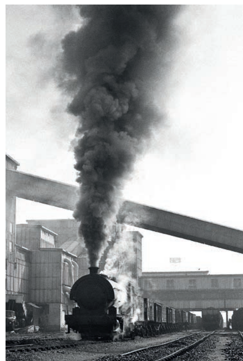
RSH outside cylinder 0-6-0ST No. 23 blasts out from under the washery at Bates Colliery on June 25, 1969.
