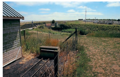
The planned extension is set to cross the stream and run to the trees in the distance, before swinging right into the car park. GARETH EVANS
