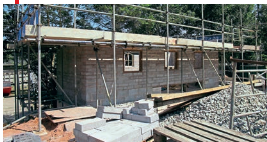
The exterior brickwork of the Corwen Central signalbox. ALL IMAGES: GEORGE JONES
