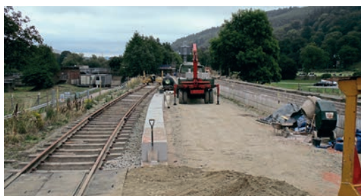
The platform 1 wall construction with gap for level crossing access.
