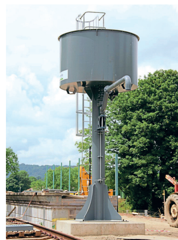
The new water tower installed at Corwen Central. GEORGE JONES
