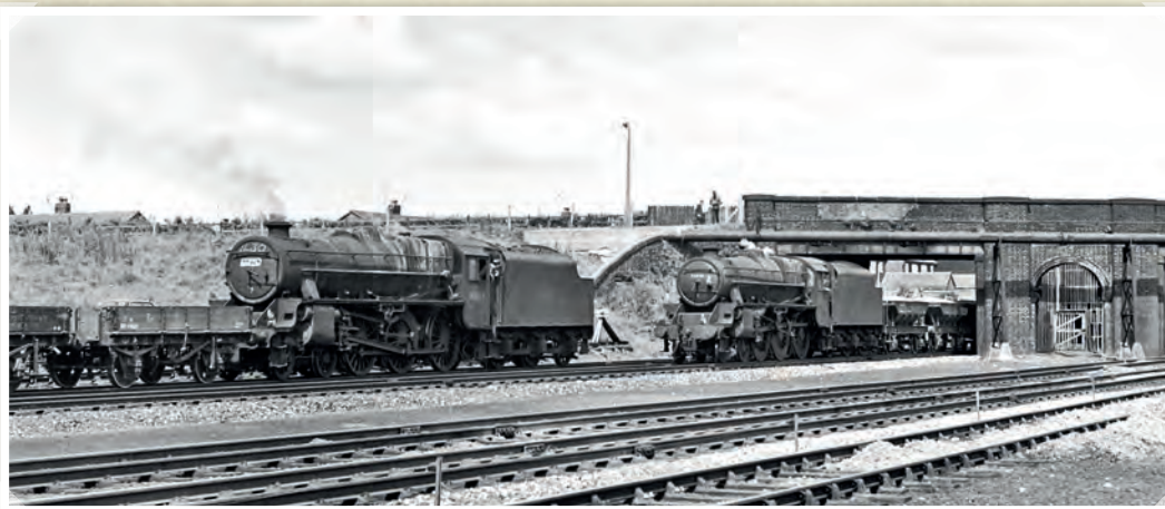
Carnforth's LMS 'Black Five' 4-6-0s Nos. 44874 and 45231 meet near Farington Junction, Preston on August 1, 1968.
