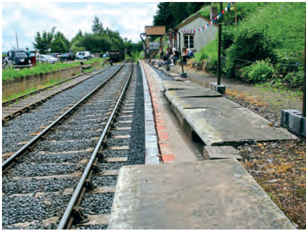
Above: With the brickwork almost complete, the focus is now on casting the edging stones to finish the platform edge, for which £8,000 still needs to be raised.
