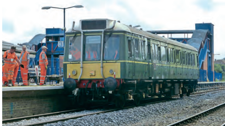
Class 121 'bubblecar' No. W55023 carried out a gauging run to the new platform 4 on June 1. CPRR
