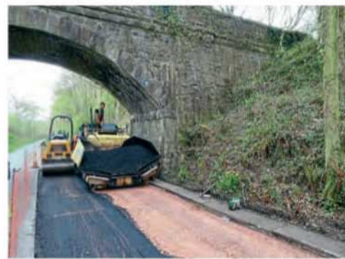
Work on the creation of a new trackbed for the heritage railway at Torrington alongside the existing Tarka Trail long-distance cyclepath which was laid on the formation of the original line. TVR
