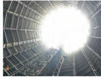
The scaffolding erected inside the Great Northern Shaft to allow repairs to take place. G BICKERDIKE/NETWORK RAIL
