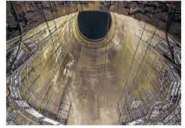
The top of Kilsby Tunnel's Grade 2 listed Great Northern Shaft seen after the repair project began. G BICKERDIKE/NETWORK RAIL
