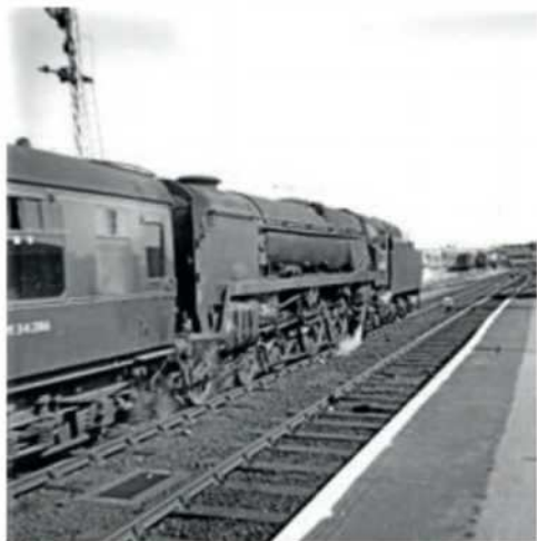
SR rebuilt West Country Pacific No. 34001 Exeter on banking duties at Poole in July 1966.
