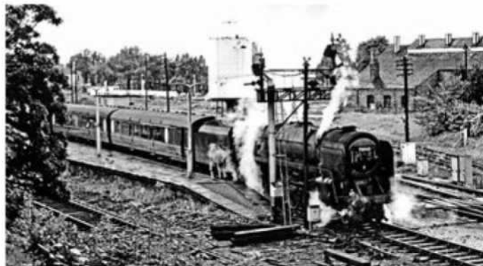
Britannia Pacific No. 70045 Lord Rowallan at Cheltenham Malvern Road station on September 4, 1965. In the background is the former Malvern Road shed, which went on to become a timber store for builders' merchants Travis Perkins, and which was demolished last year. DAVID ALDRED/GWR
