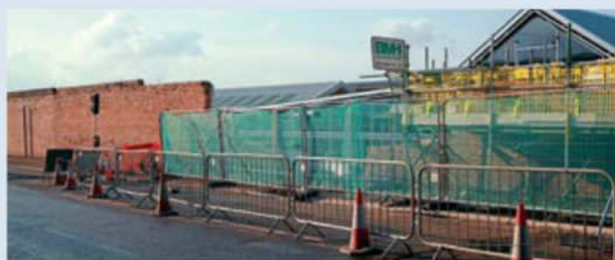
Demolition of the 135-year-old Wolverton Wall began in February. However, the Judicial Review may yet throw a lifeline for the historic works. PHIL MARSH
