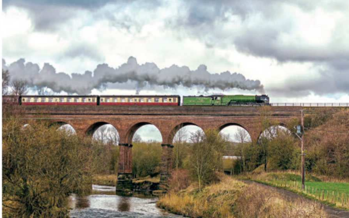
LNER A1 Pacific No. 60163 crosses the Roche Viaduct near Heap Bridge on the East Lancashire Railway on March 29.
