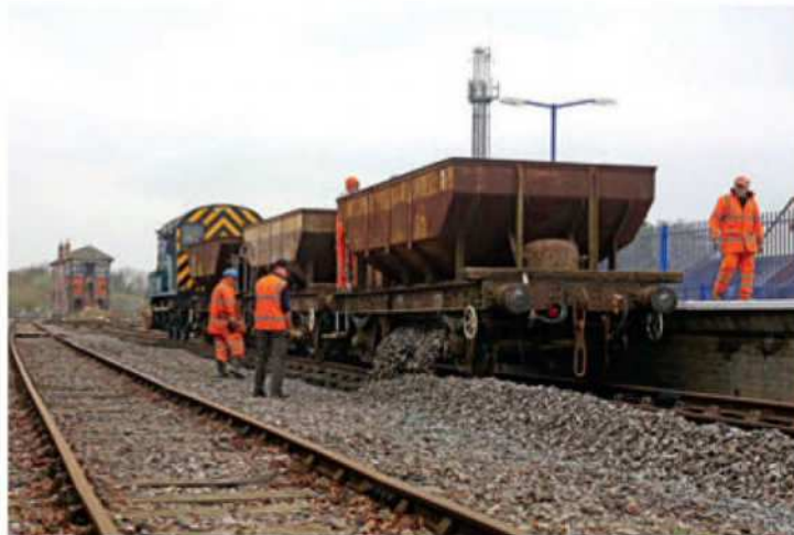
Ballast being dropped on the day that the first train ran into the Chinnor & Princes Risborough Railway's new platform at Princes Risborough. ANDREW ROYLE
