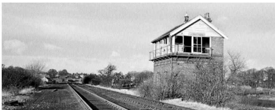
The derelict Alnwick East signalbox and the partially-lifted second track.
