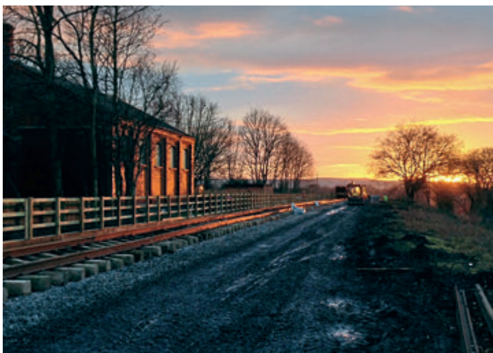
The connection in place: the unballasted line past the former Broadway goods shed on December 23. NIGEL BLACK/ G/WR
