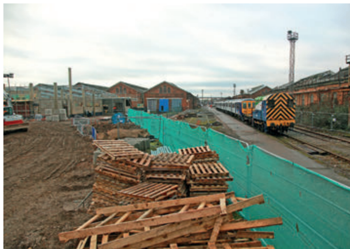
Wolverton Works disappears from view behind the new Lidl shop as Class 319 EMU 319386 is shunted by Class 08 No. 08629 on December 20. PHIL MARSH
