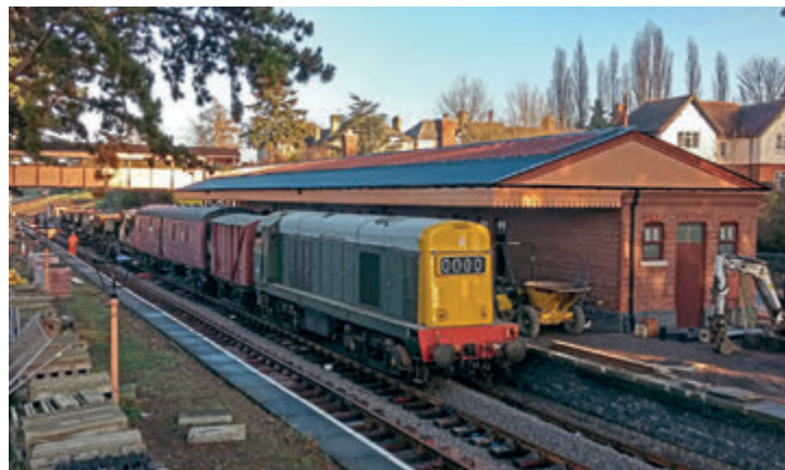
Class 20 D8137 heads a permanent way train laying ballast at Broadway station on December 23. G/WR
