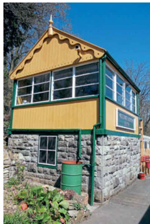
The restored Midsomer Norton signalbox on April 14, 2015:
