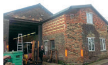
The north end of the Redhill locomotive shed. REIGATE SOCIETY
