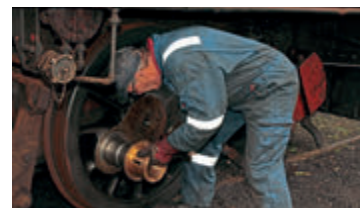
One of the bearings being fitted to Class 03 D2178. GWILI RAILWAY
