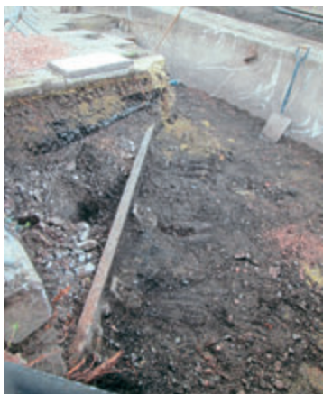
A rail from the Totnes Quay branch uncovered during flood prevention works. TOTNES TIMES
