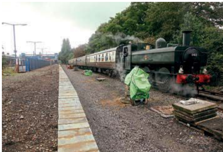
An interchange in the making: on-loan GWR 0-6-0PT No. 6412 and its train from Chinnor stands in the area at Princes Risborough station leased from Network Rail opposite the new under-construction platform for the heritage line. PHIL MARSH
