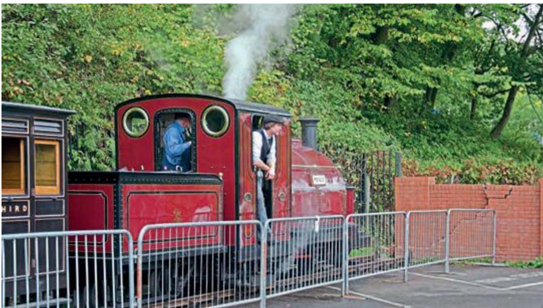
This brick wall came off worst when it was struck by the front coupling of the Ffestiniog Railway's England 0-4-0STT No. 2 Prince at 1mph while the locomotive was giving a demonstration at the Engine House visitor centre at Highley on September 23, during the Severn Valley Railway's autumn steam gala (News, pages 32-33). JOHN TITLOW
