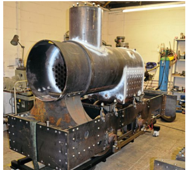
Right: The Decauville locomotive taken on May 26. The firebox wrapper/boiler barrel has now been fitted, along with the inner firebox and front tubeplate. At this stage the cylinders and steam chests were still to be attached, although work on these items was well advanced.
