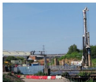
The work in progress to install piles for the new bridge at Loughborough, as seen on June 17. ROBIN JONES
