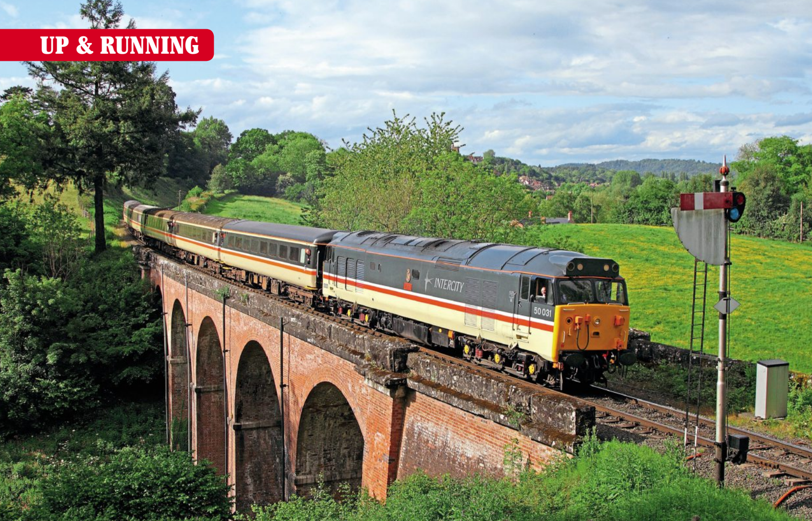
Class 50 No. 50031 Hood crosses Oldbury viaduct during the Severn Valley Railway diesel gala. JAMES HAMILTON
