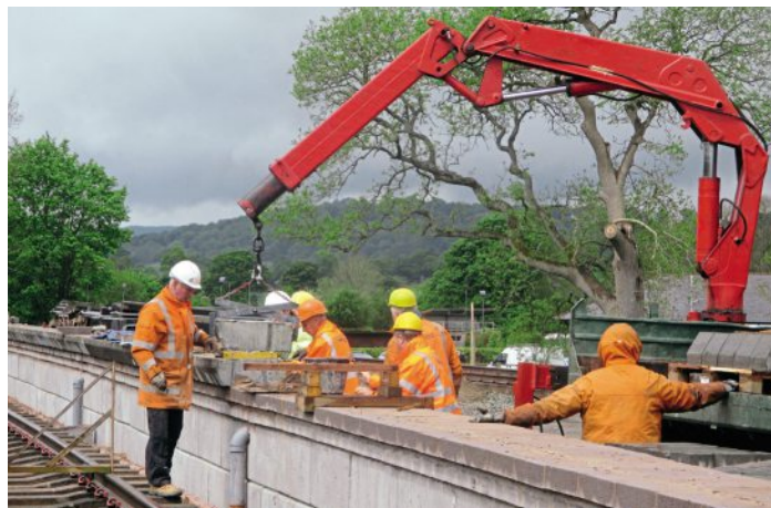
The volunteer workforce tackling the oversail blocks on Corwen Central platform 2. GEORGE JONES
