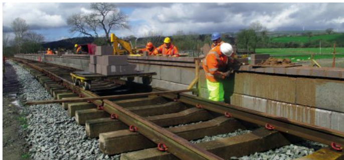
A platform wall taking shape at the new Corwen Central station. GEORGE JONES/LR
