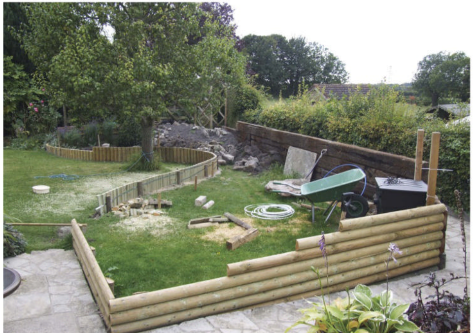
September 2009, construction well underway. Once an unruly hedge had been cut back, it opened up another 4 or 5ft of available space, which allowed a path to be laid at a lower level. Building up a wall of sleepers gave the main station (Teslin) a working height of about 4ft. The lower levels make use of 4" half-round timber, either longitudinally or in a 'log-roll' form.
