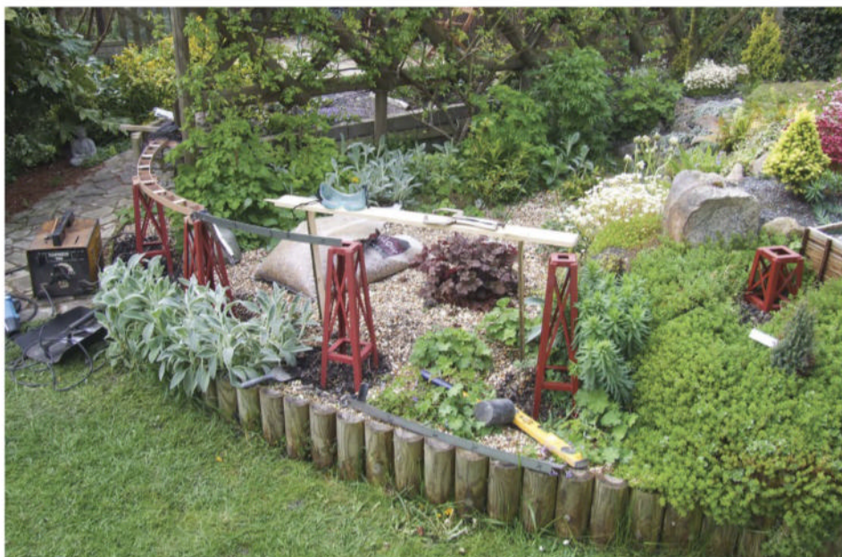
The last major construction project before the line could be completed in 2012 was the viaduct across Glacier Valley, as this area became known. Made from steel angle and strip. I welded the towers up before setting them in the ground, and then welded steel strip to the towers to support the track.
