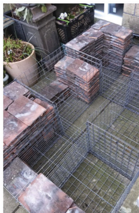
Filling the gabions with the derelict, century-plus-year-old tiles from the roof at the in-laws. Nice to be able to upcycle and re-use these, and save them going to the tip.
