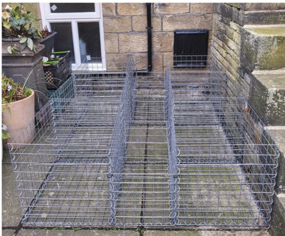
The gabions being built; a nice strong foundation for the railway and quick to build.
