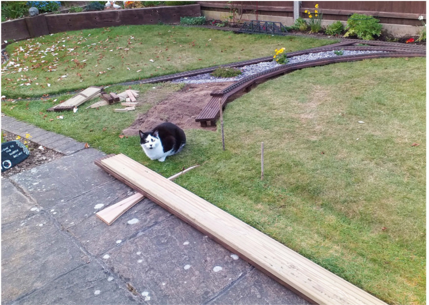
Construction starts, with the foreman looking on.
