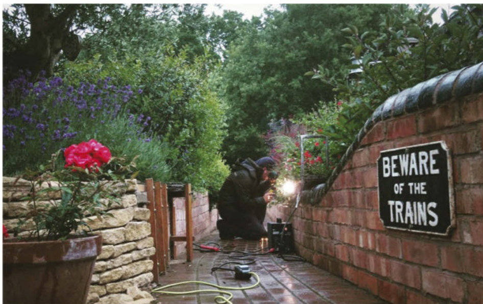
Some last minute welding to prepare the bridge for use.
