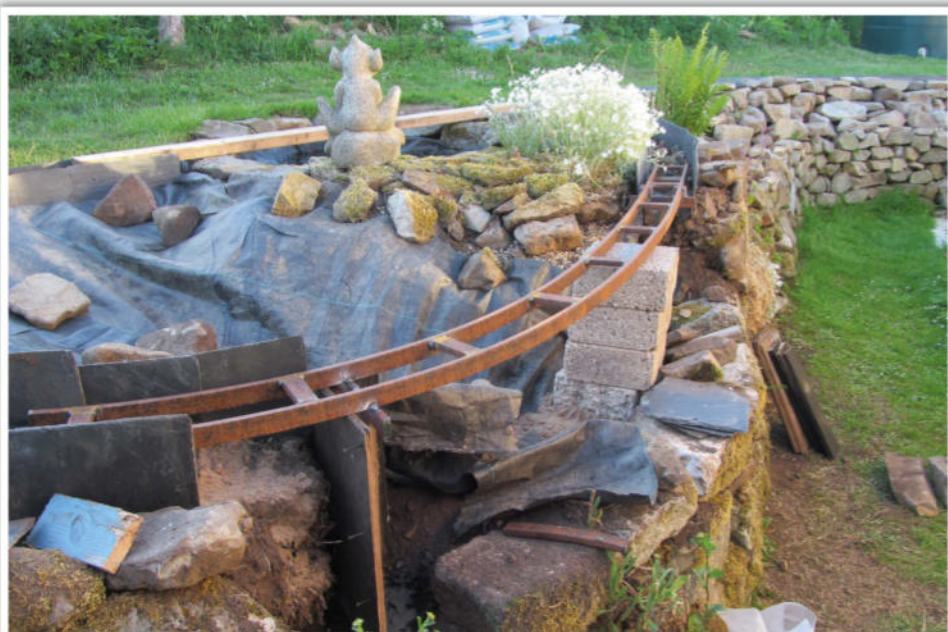
Bridge construction. The main structure is a welded framework of the 30 x 12mm steel bar we use as rail on our 7 ¼ inch gauge railway. At this stage, the metal T-shaped supports are concreted into the ground prior to being encased in cast concrete to form the abutments at each end of the bridge. Much later, a couple of metal trestle supports would be added to improve the look of the bridge, but they are completely unnecessary structurally.
