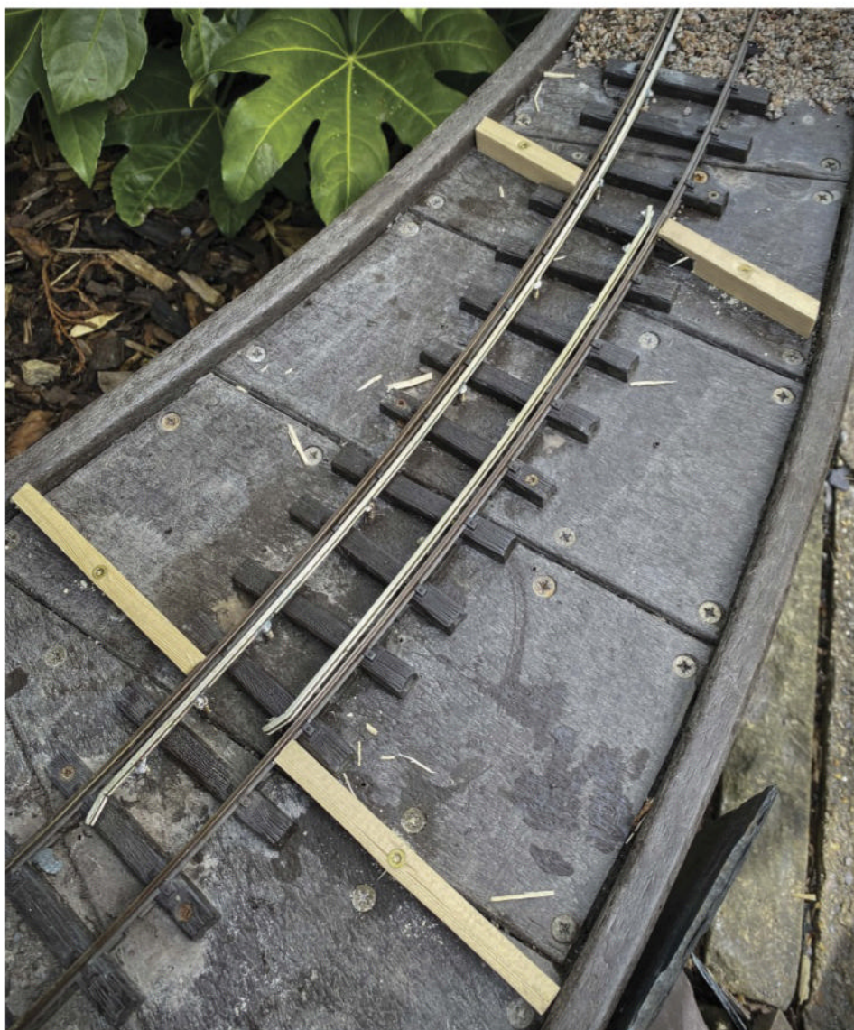
Shuttering made from lengths of wood in place before the mortar mix is poured for the crossing.
