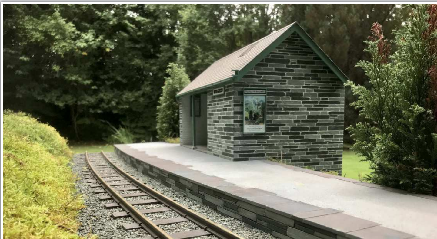
Completed station building and landscaping section.
