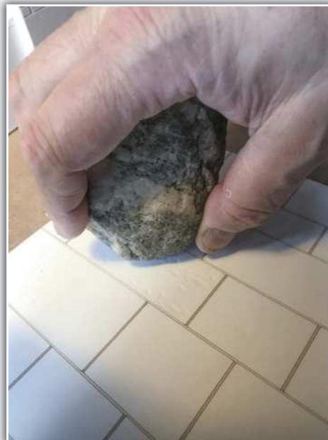
Distressing the surface of the slab flooring prior to carving the stone detailing.
