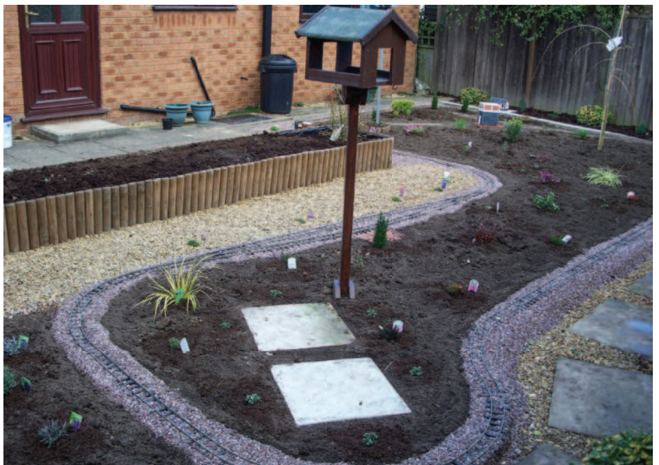
A firm trackbed using bricks and ballasted with horticultural grit. The middle of the railway was filled with top soil before the planting of new plants.
