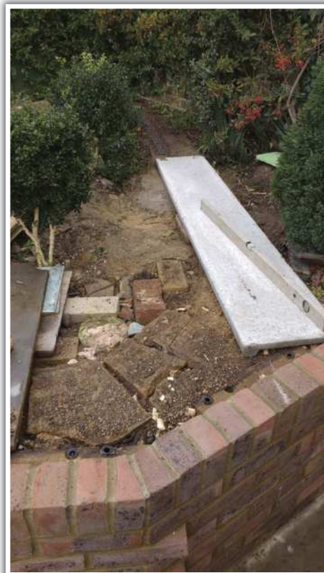
Replacing the viaduct with concrete gravel board.
