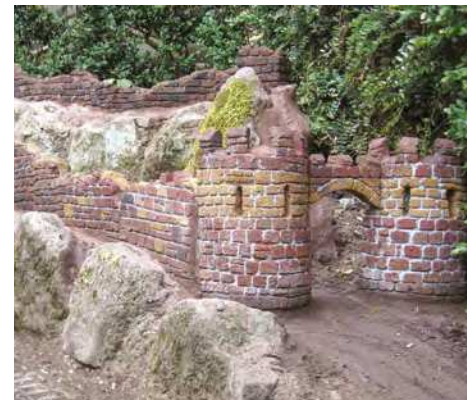
The sections were then assembled – a 3:1 (sand:cement) concrete mix being used to fix them to the foundations and exterior PVA used to join the sections together.
