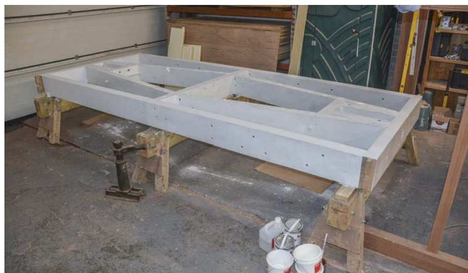
This illustrates the current state of the 12" to the 1' project I'm involved with, an extensive rebuild of van G1 of 1872 by the Isle of Man Steam Railway Supporters' Association. The joinery for the underframe is now all but finished and makes a good reference for modellers.
