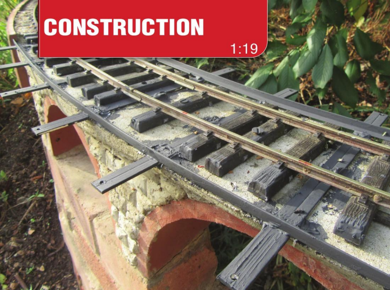
1/4in wide Plastikard angle strip was glued to the deck to contain the track ballast.
