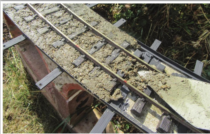
Ballast was a mixture of five parts sharp sand, one part O scale granite ballast, and one part cement. This was applied with a small trowel and cleaned off the sleeper tops and rail sides with an old toothbrush and screwdriver before the cement had set.
