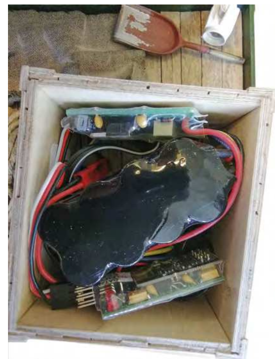
The electronics stuffed into the crate. There's not much spare space in here!
