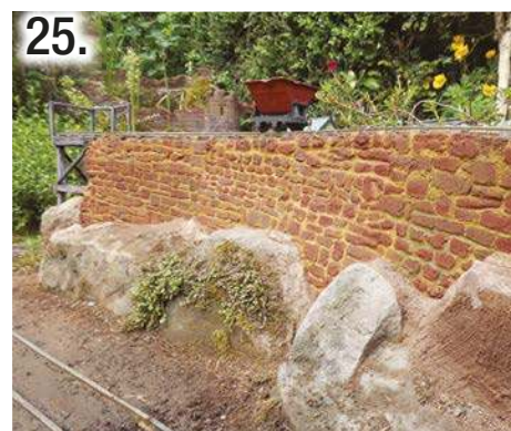
25. After careful thought, I decided that the hoppers would be loaded from a two foot gauge (32mm) feeder railway on an embankment. This was cast in dyed concrete using wooden formers with mortar courses lined out with hot-glue to act as a mould.
