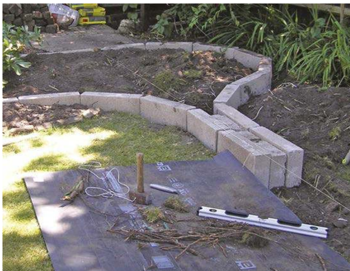
The entry to the embankment from the ground level, note the master level string, spirit level and Grandmother's lump hammer.
