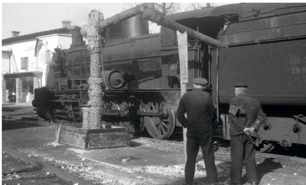
Left A rare picture taken during the 1950s in Planica, the Yugoslav border station facing Fusine – Laghi in Italy. The JDŽ class 28 is a twin of the FS Gr.476 (visible in the Italian picture above). It is interesting to note how the water column has been wrapped in a layer of rope to protect it from the terrible winter cold in this area. Photo: archive Muzej Noveiške Zgodovine Slovenije.
