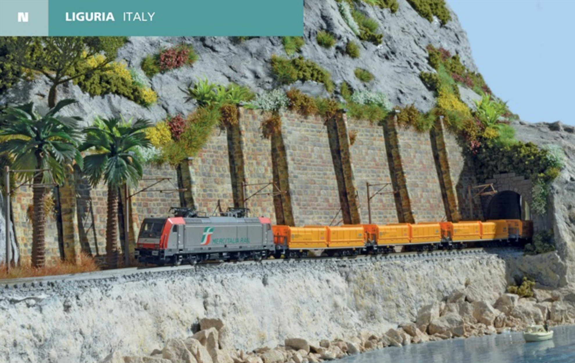
Left An E.483 rolls slowly by with a load of side-discharge ballast containers.
