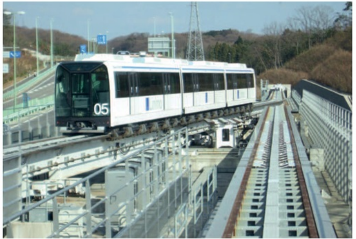
Above New technology 2. Magnetic levitation transit system 'Limino' opened for the Expo in Nagoya in 2005.
