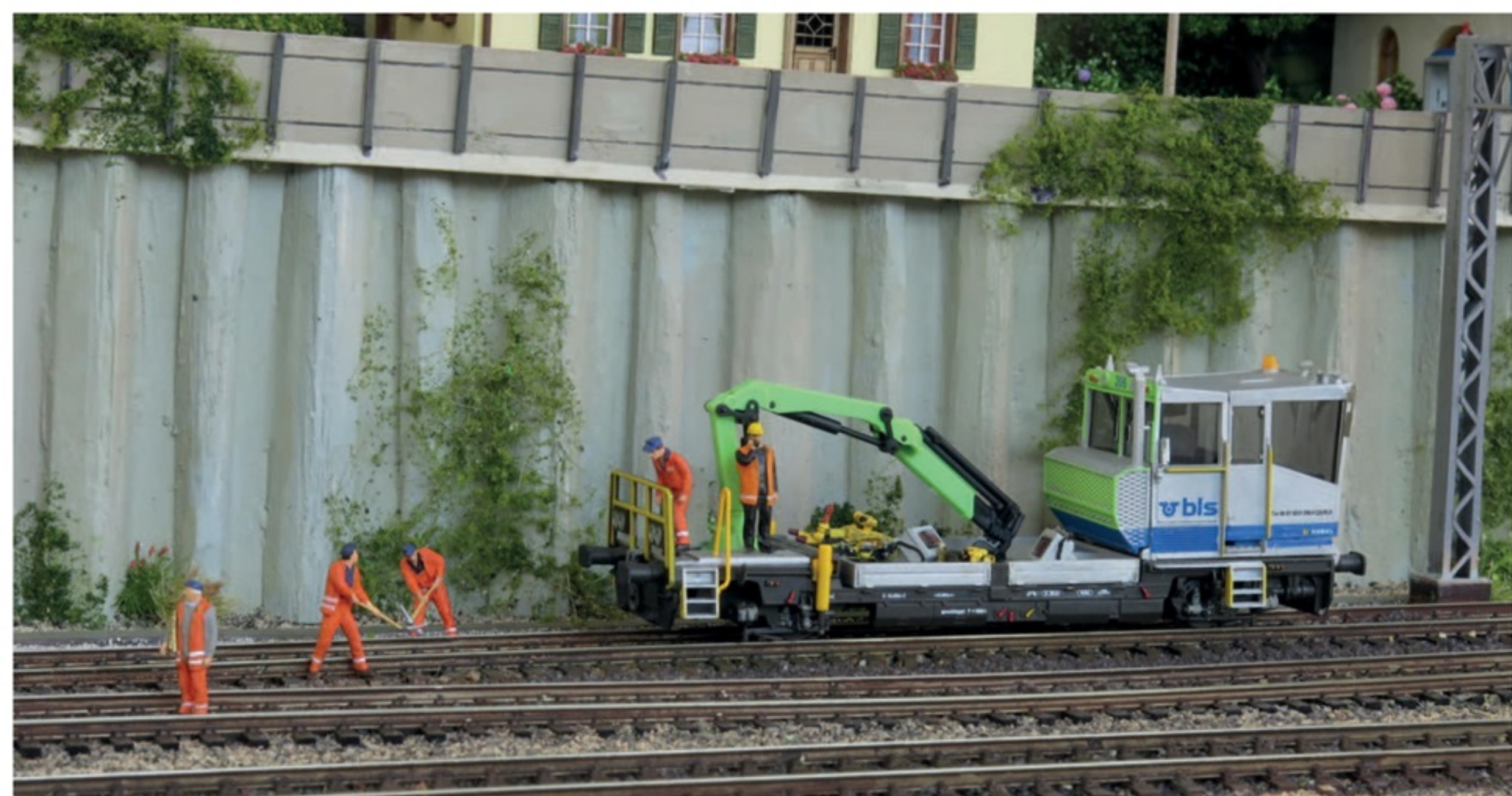
Above left BLS 420 504 stands below the retaining wall at Spiez station receiving attention.
