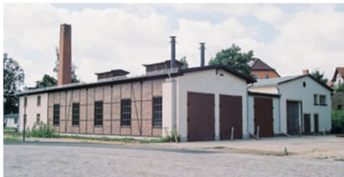
Left The former loco shed and workshop at Wilsdruff, restored as the centre of a heritage project, in August 2010. Since then much progress has been made and track has been relaid with the aim of having a working line as far as Wilsdruff Haltepunkt.
