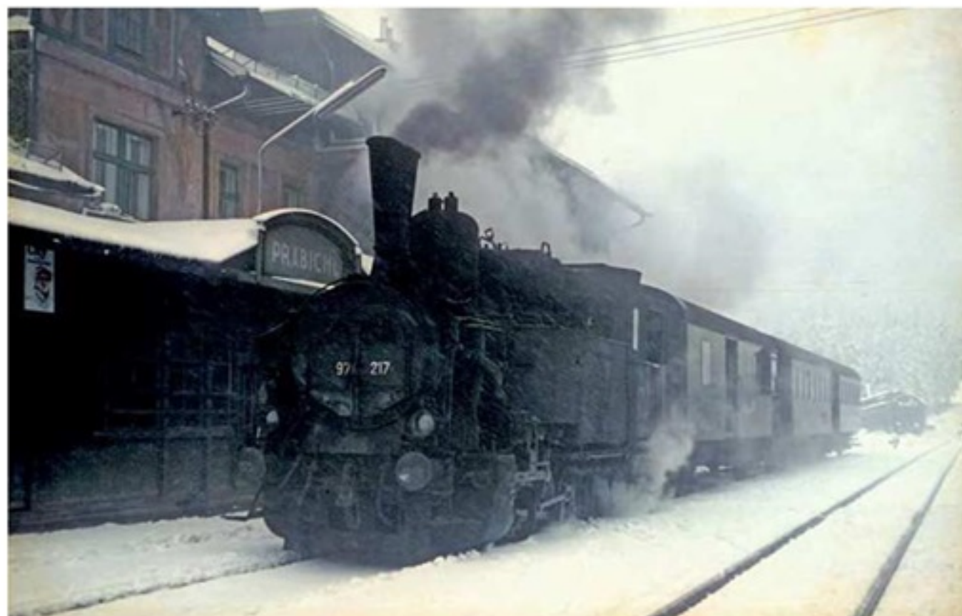
Below 0-6-2RT 97.217 in the snow at Präbichl station. 8th October 1974.
