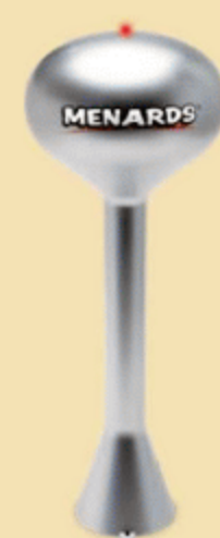
LIGHTED WATER TOWER
