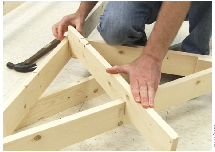
The rounded corner design found at one end of the layout required special framing formed by making 45-degree cuts on the ends of the 1 x 4 pine lumber components.
