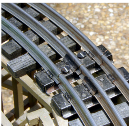
FIG 6. Extra railroad ties (two ¼-inch square wood pieces glued side by side and painted flat black), add the finishing touch to the bridge deck.
