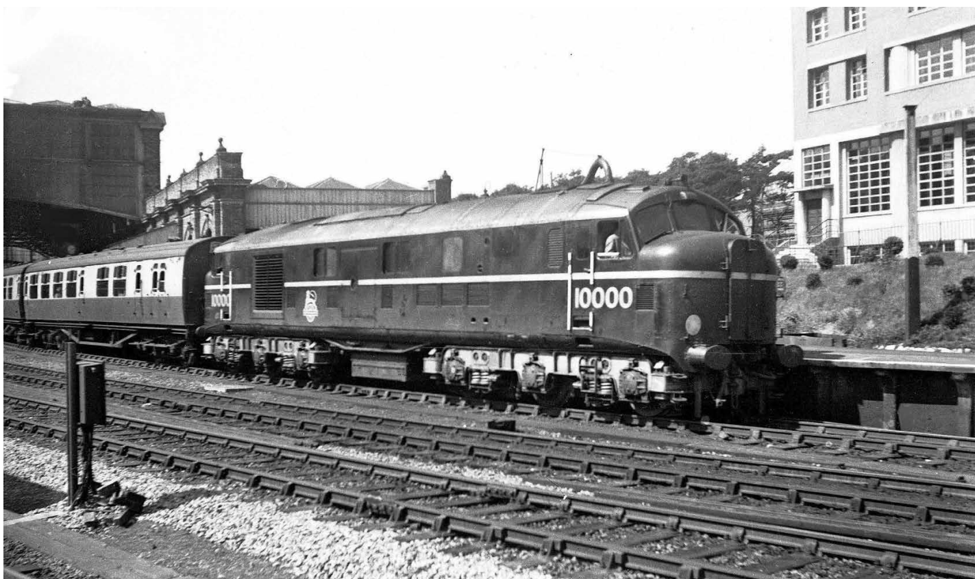
Co-Co 10000 in Bournemouth on May 3rd, 1953, after its transfer from the London Midland Region to the Southern. During its stay on the SR, this locomotive was overhauled and repainted in Brighton Works and received a smaller BR crest.
