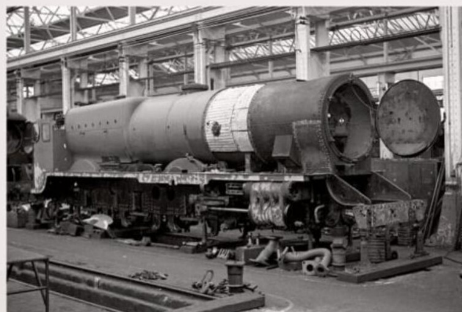
Anatomy of a Nelson as 30857 undergoes an overhaul at Eastleigh Works. A J Wigley/Colour-Rail.com
