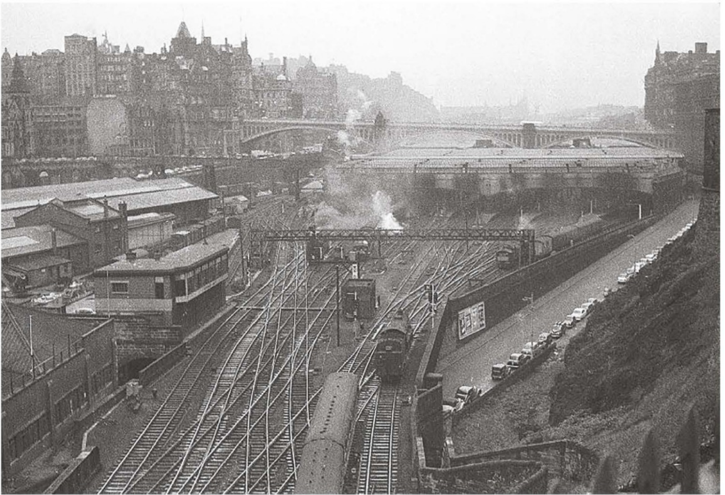
Edinburgh Waverley station complex from above the Calton Tunnel portals. P Elmslie
