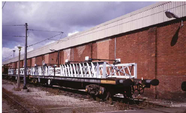
Also recorded at South Gosforth in August 1987 were the two PFAs, MA1 and MA11, which had been fitted with frames to carry cable drums. DAVID RATCLIFFE
