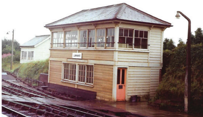
Liskeard signal box; the first mechanical signal box to be encountered in Cornwall. August 22nd, 1978.
