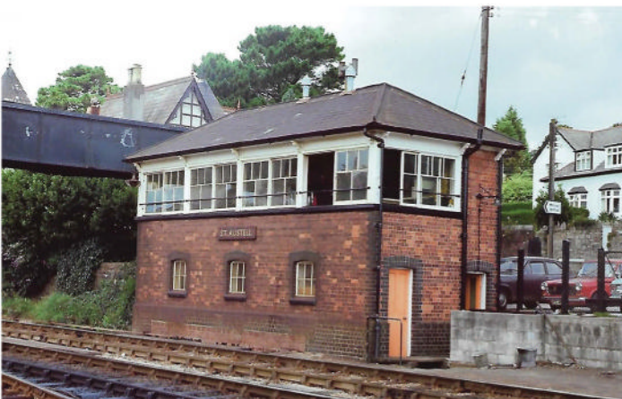
St. Austell signal box on August 18th, 1978.
