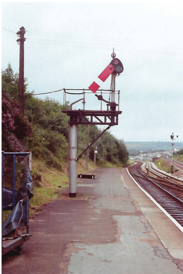
Liskeard down main platform starting signal. The Up sidings are to the right.
