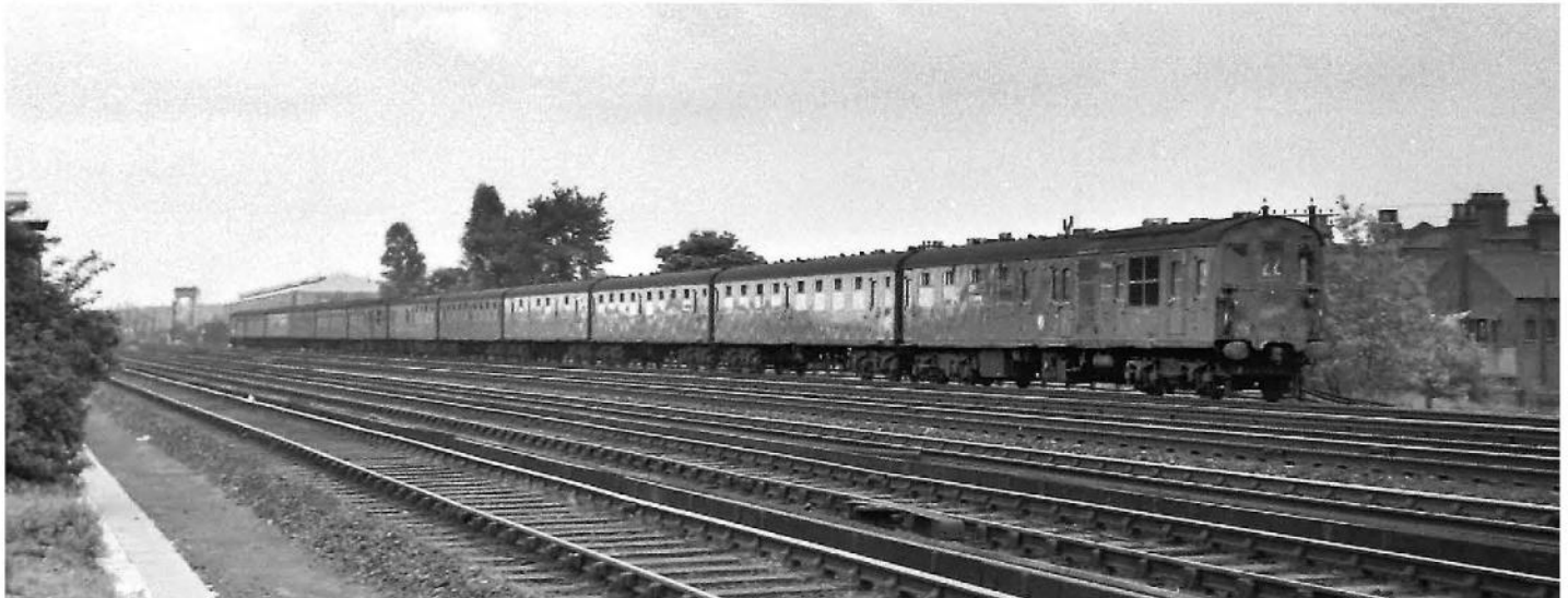
The Hasting DEMUs began to replace steam locomotive-hauled services between London Charing Cross and Hastings as early as 1957. In this 1960 view, a pair of six-car units passes Hither Green at speed on an up service. The leading unit is a later one on long underframes, whereas the rear unit is an earlier short underframe unit with lower seating capacity. These trains were geared for 90mph. COLIN BOOCOCK
