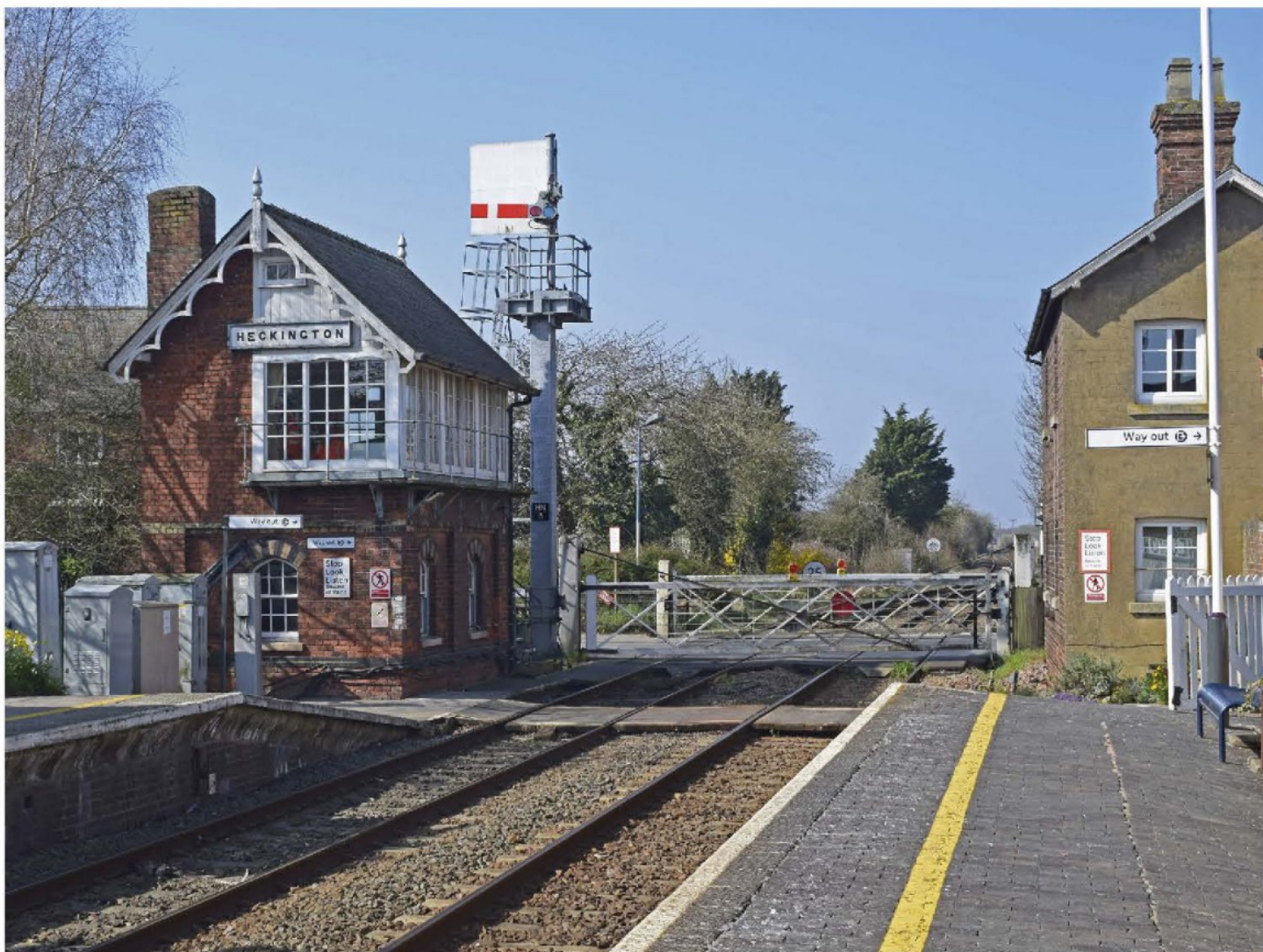
Traffic at Heckington station in Lincolnshire is controlled from a GNR signal cabin of 1876 (grade II listed) with conventional level crossing gates and a modern upper-quadrant home signal. Robustly constructed of galvanised steel posts, ladder and landing, the unit is equipped with a rectangular sighting board.
