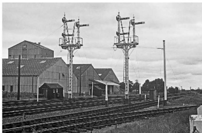
These elegant upper-quadrant junction signals once guarded the eastern approach to Sleaford station, being mechanically-operated from Sleaford East signal box built by the Great Northern and Great Eastern Joint Railway in 1882. With lattice lower and upper posts, these units are typical London North Eastern Railway (LNER) in design, supplied by McKenzie & Holland. Note the tall ancillary posts supporting numerous guy ropes to stabilise the signals. This image was captured in 1969, another undated reference indicates distant arms on both right-hand, lower posts.
