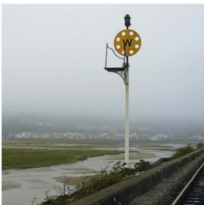
Disc signals once acted as auxiliary signals throughout the Ffestiniog railway system. This unit situated on the Cob, close to the junction with Boston Lodge works, acts as a fixed distant, warning drivers of the possibility of the next signal being set at danger. Often positioned at the approach to a station, a working version would be operated by a capstan linked by an axle-rod.
