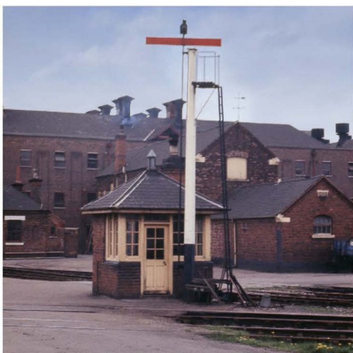
Installed by the Midland Railway, crossbar signals became a familiar sight throughout the Bass brewery railway system at Burton upon Trent. This unit, guarding a level crossing, survived in use until the demise of the line circa 1970. At the foot of the post, the capstan and turning mechanism are discernible, also the narrow vertical shaft connecting it to the crossbar and lamp.
