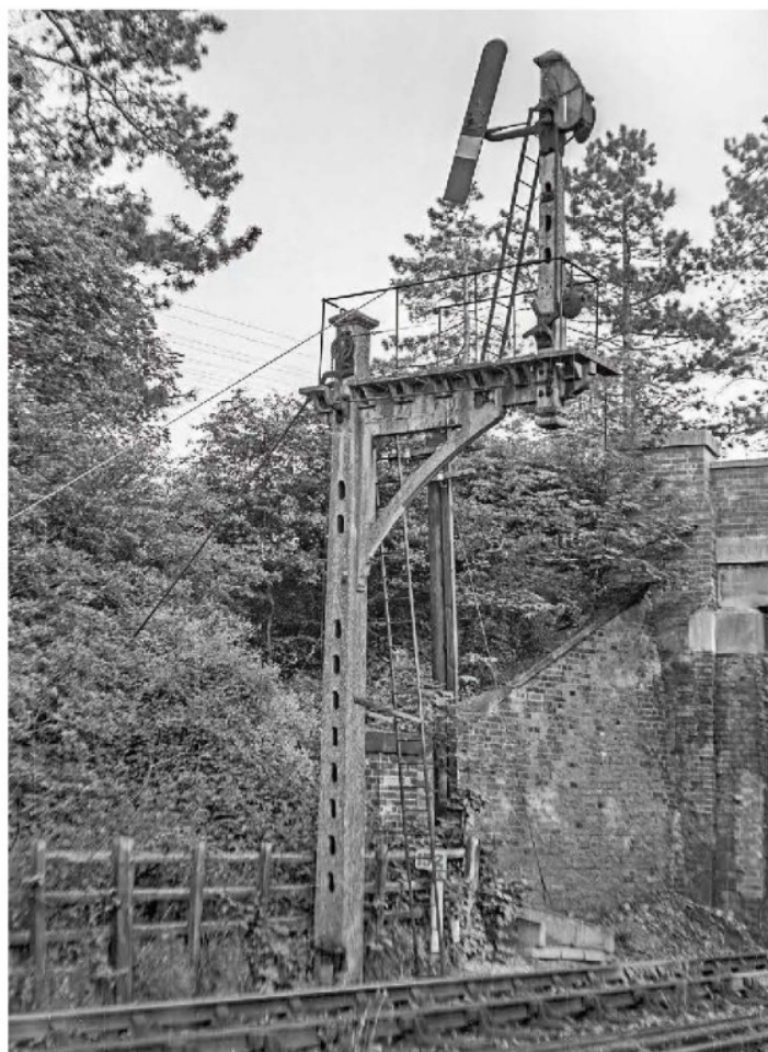
The GNR favoured the somersault type of signal following a serious accident at Abbots Ripton in 1876. On that occasion, an arm failed to return to danger due to the weight of ice formed on it. Situated at Etwell on the ex-GNR Derby-Egginton Junction route, both posts and bracket are cast in concrete. Apart from reducing the cost and weight, the oval holes in both posts lessen wind resistance and make handling easier during assembly. Note the balance bar and weight at the bottom of the bracket post are linked by wire and pulleys to the signal box. Photograph by Phil Waterfield.
