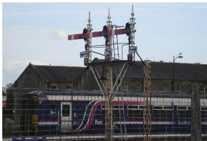
Observed at Stirling in 2007, prior to a signal improvement programme, this triple junction unit was controlled from 'Stirling Middle Box'; a type N2 cabin, its original lever frame by Stevens GNP, it was built by the Caledonian Railway in 1901. Most semaphores at this station consisted of lattice posts with upper-quadrant arms, but one lower-quadrant type survived until 2000. Note a second post to stabilise the main unit with what appear to be rigid links.
