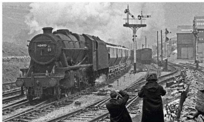
The MR junction signal at Peak Forest on that railway's main Derby-Manchester line is a classic example of a product of the Derby signal works. The right-hand, taller, lower-quadrant arm gives right of way to the passing limestone train, while the left-hand controls access to any traffic from the sidings. Note the signals to the right, in the sidings, appear to be upper-quadrant and may have been installed later.
