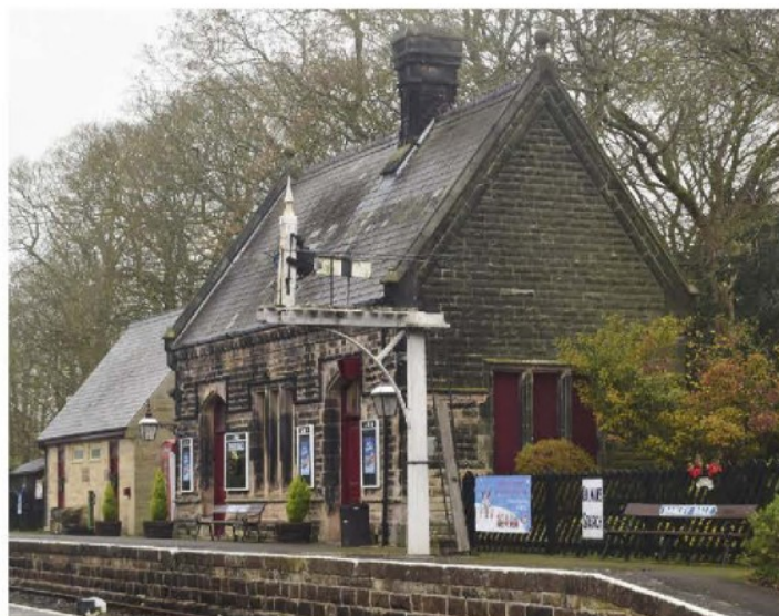
At Darley Dale heritage station, the signalling equipment has been sourced from other areas in the Midlands. Clearly of MR origin, this upper-quadrant arm, cantilevered from a timber post, replaces a taller unit with a single post that occupied the same position in earlier days, on the southbound platform. Note that due to the siting of this signal on a platform, the access ladder has been made secure by attaching a plank over its rungs, and the control rodding needs to be out of public reach.
