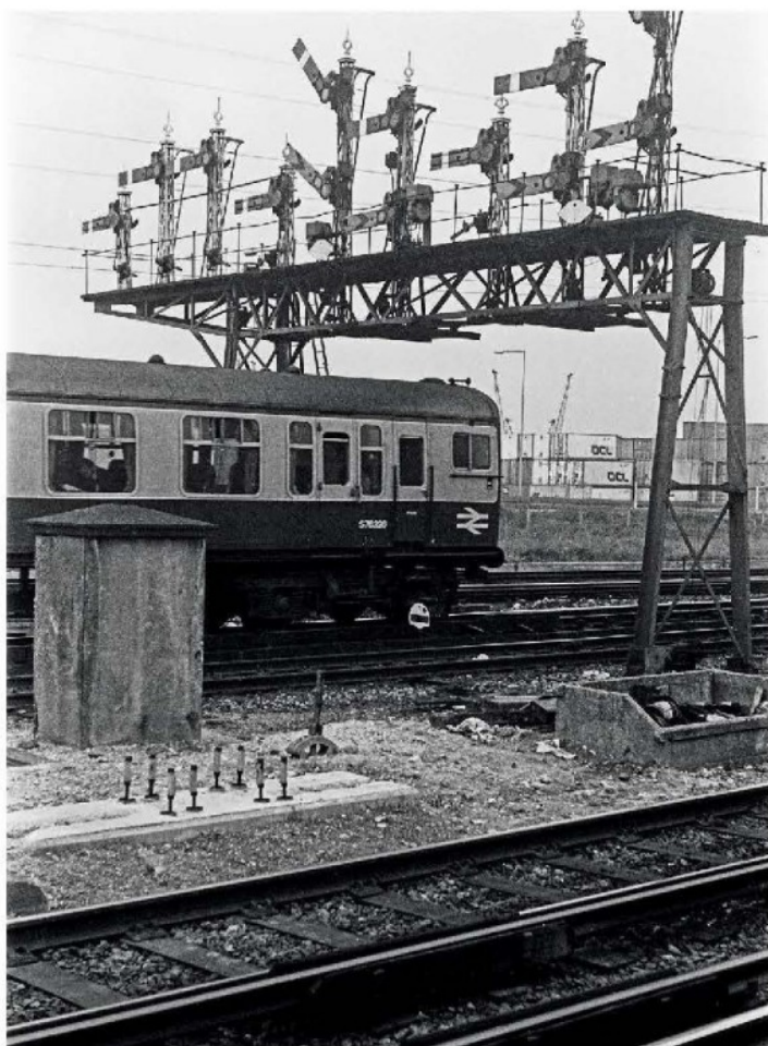
This signal gantry, with lattice style structure and upper-quadrant arms, controlled movements at the western end of Southampton Central station. Originally named Southampton West when opened by the LSWR in 1895, its name changed to 'Central' in 1935 following being enlarged by the SR. The signal gantry would have been erected at that time, lattice construction being commonplace on the SR. Present-day images reveal two gantries of modern construction supporting colour light equipment and the defunct art-deco style 'Southampton Central' signal box.
