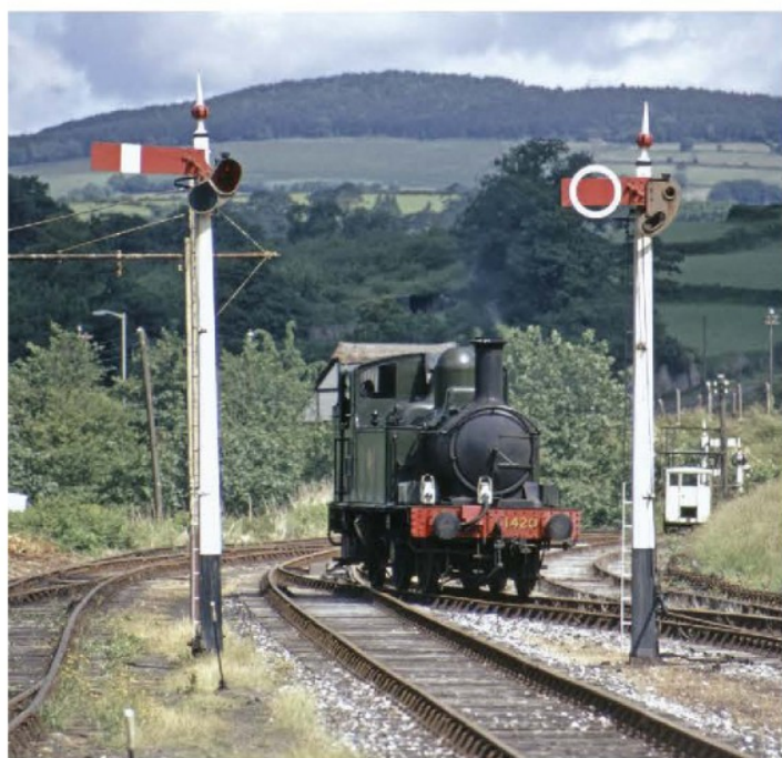
Captured at Buckfastleigh in 1969, these two early GWR lower-quadrant signals have tapering timber posts and cast finials. Such posts measured 0.15m (6in) square at the top and tapered at 1ft in 5in to the bottom, a process carried out in the planing shop at the company's signal works at Reading. The white ring attached to the arm of the right-hand unit indicates passage from a siding onto a main line; a similar example remains at Buckfastleigh station as a heritage feature.
