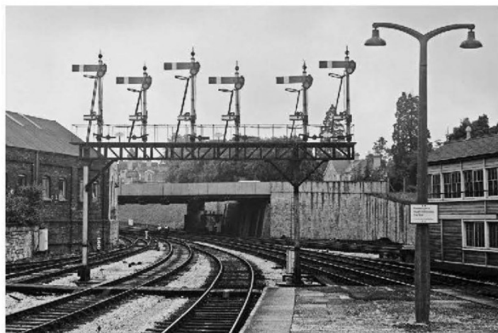
This signal gantry consisting of tubular posts and lattice span controlled some of the movements at the west end of Newton Abbot station. To the right of this image, captured in the summer of 1982, 'Newton Abbot West', GWR (type 28C) signal box, is visible. Opened in 1927, it is likely that the signal gantry with lower-quadrant arms would have been commissioned at that time. Each of the six posts carries a home arm and 'calling on' or 'shunt arm', also on the span, three white diamonds are displayed to inform locomotive crews that there is no need to call the signaller if held at that signal. Re-signalling of the whole station area occurred later, during the 1980s, replacing this gantry and others. One such structure is now preserved at a nearby location.
