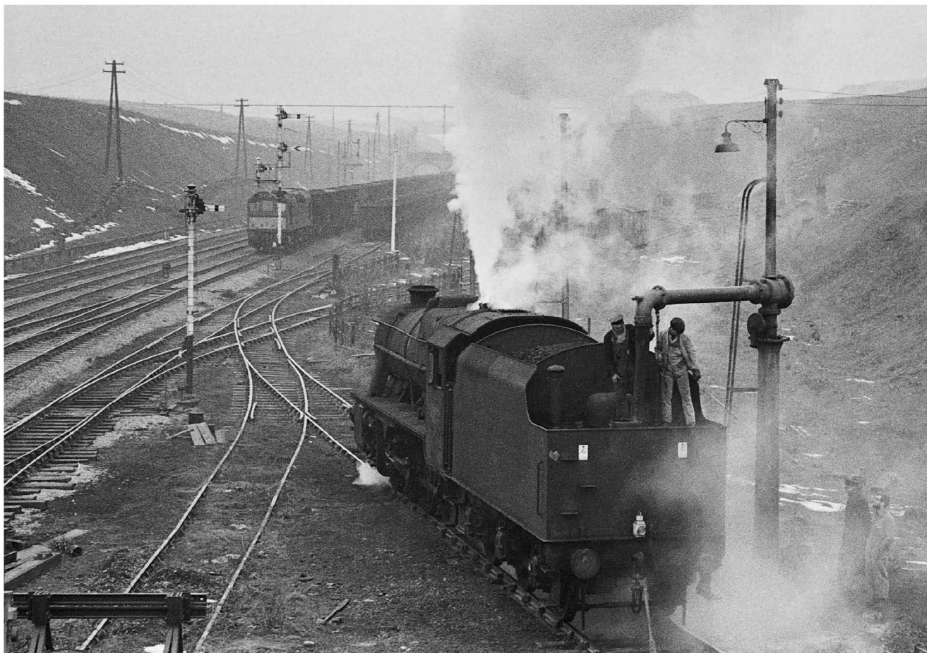
This water crane, adjacent to a turntable, facilitated locomotives handling limestone workings at Great Rocks Junction on the ex-Midland Railway's Derby-Manchester route, to the east of Buxton. In March 1968, the two operatives standing atop the Stanier class 8F's tender attempting to align the bag with the tank filler port, rely on their two colleagues on the ground to turn off the supply when the tank is full to avoid being soaked by a splash-back. A water tower consisting of a rectangular tank mounted on a low concrete base maintains water pressure from its position on a neighbouring hillside.
