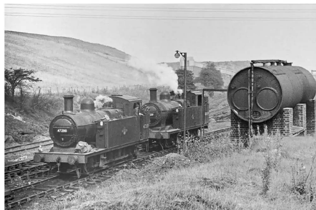
This horizontally mounted water tank at Williamthorpe colliery, accessed via Avenue Sidings on the Erewash Valley line, near Chesterfield, probably in an earlier life served as a boiler. A not uncommon use for such an item on industrial railway sites. Pumps were possibly housed below the tank, the supply pipe is identified as connecting a number of ports on top of the tank. This 1967 image features two ex-LMS Jinties contracted by the National Coal Board from British Rail, based at Westhouses MPD.
