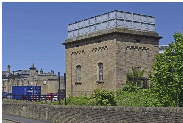
The Grade II listed, Keighley water tower is an example of a Midland Railway installation; erected in 1883, the tower was built of dressed stone and the tank comprises two levels of cast iron sections. Its architecture is typical of many MR structures, particularly to be found on the Settle-Carlisle route. Sited on the platform used by the Keighley and Worth Valley Railway, plans are afoot to use the redundant building as an information centre.
