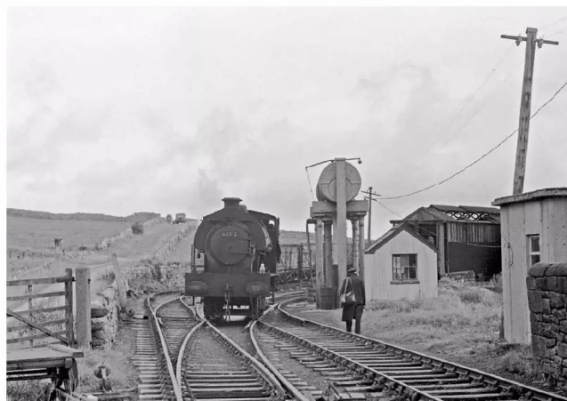
The cylindrical tank mounted on timber blocks, supported by what appear to be cast iron columns, supplied water to locomotives working the Cromford and High Peak Railway at Middleton Top. Along the line at Sheep Pasture Top, a similar water tower with a larger capacity tank served the same purpose, drawing its water from an adjacent reservoir. Sheep Pasture Bottom also had a water tower – a rectangular tank mounted on a timber frame and fed from a hillside spring. Water was a scarce commodity in the High Peak region; contracted to supply water to various industrial sites, farms and households, this business enabled the railway to survive until 1967, delivering the liquid in ancient ex-locomotive tenders.
