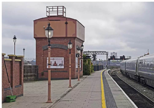
When steam returned to Birmingham Moor Street station, the long-gone locomotive water supply needed to be resurrected. Restoration sympathetic with the GWR styling of the station originally opened in 1909, occurred between 2010-14. To accommodate the steam-hauled charter trains, a water tower would be required. The structure illustrated was removed from Tyseley depot and re-erected on platform 3 at what has become Birmingham's second busiest station. With brick-built tower and GWR-style tank, the structure rests comfortably with the Moor Street station architecture. A predecessor stood on columns nearer to the station throat on the opposite side of the rails, almost opposite the one-time large, hip-roofed signal cabin.
