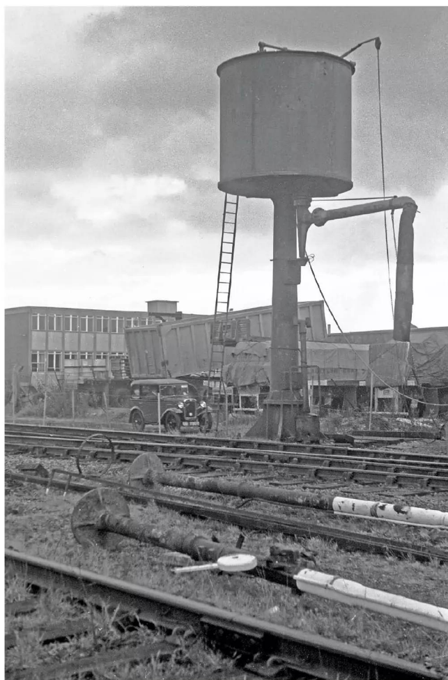
This water column on the ex-Great Central line at Loughborough, photographed in 1974 during the early months of the heritage railway, survives. The supporting column conveys the water to the cylindrical tank above. This image shows the rotating boom, bracketed from the column, from which the bag hangs. The fixed ladder enables inspection of the valve that maintains the correct water level. Note the fire devil, by the column, with tall flue, probably intended to carry heat to a higher level.
