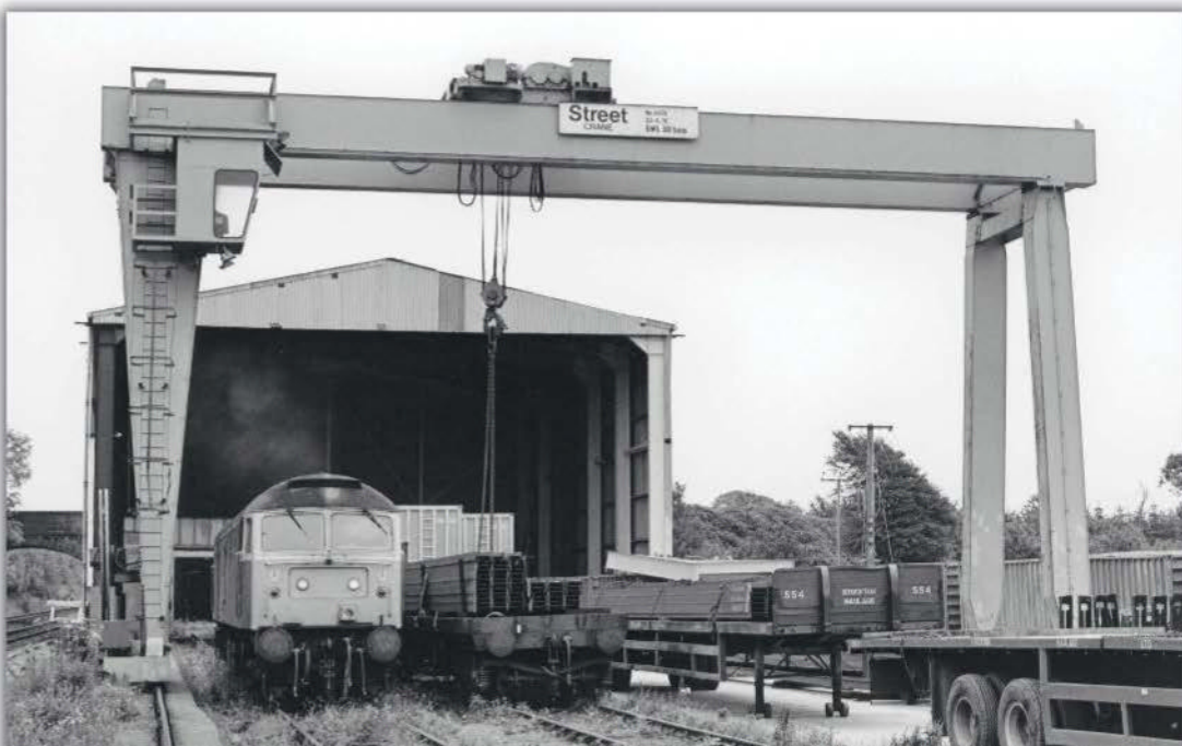
The Stockton Haulage depot at Stranraer Town handled steel for export to Northern Ireland as well as other types of freight. At its height the terminal received three trains a day, although train weights were limited by the gradients on the line between Ayr and Stranraer. The Stockton Haulage gantry crane is poised for action as 47211 waits in the adjacent siding on 25th July 1985. PAUL SHANNON
