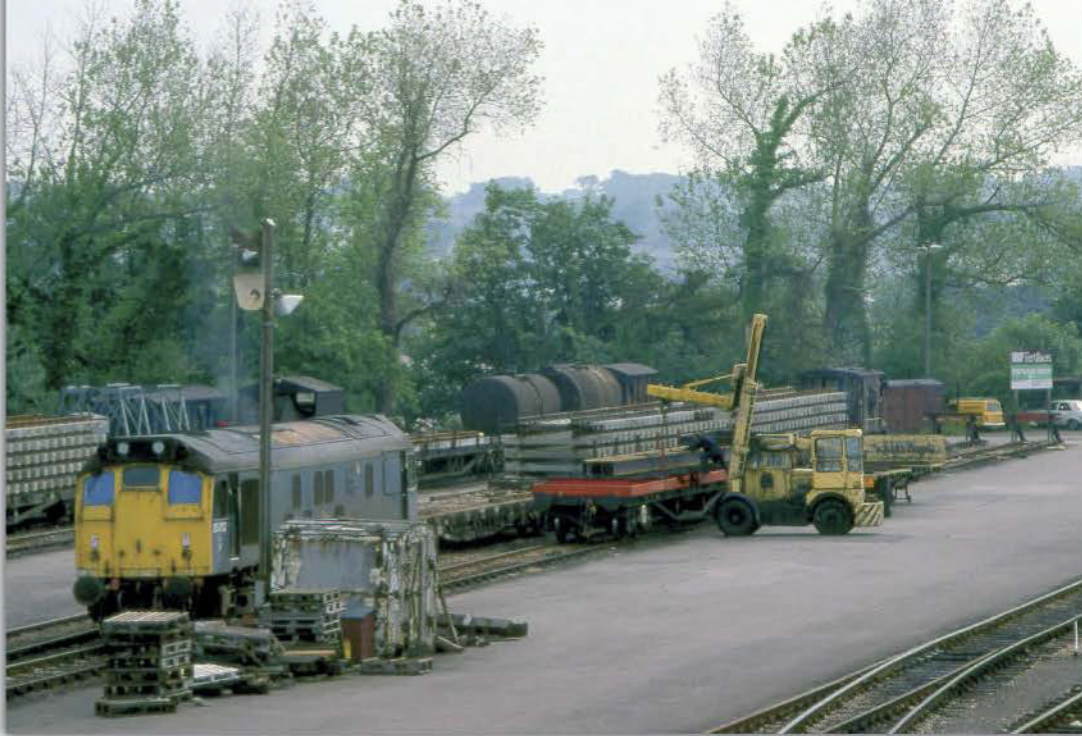
Many BR goods depots had suitable facilities for handling wagonloads of finished steel. Where no permanent crane was available, mobile equipment could be hired in as necessary. With 25052 ticking over between duties, girders are lifted from a BDA bogie bolster wagon in Truro yard on 11th June 1980. PAUL SHANNON
