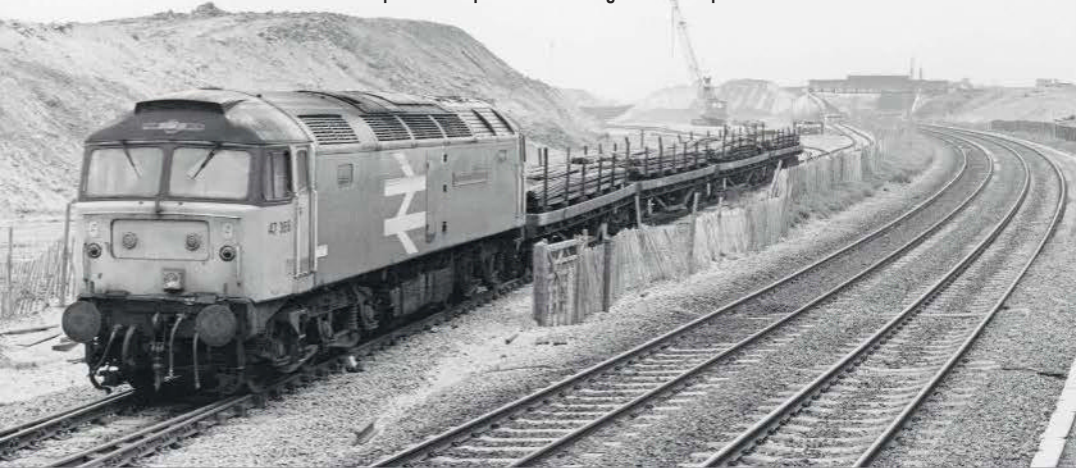
The building of the A55 expressway along the North Wales Coast generated flows of steel reinforcing bars and cement to a temporary terminal at Conwy Morfa, just west of Conwy. 47366 shunts four BDA steel carriers at Conwy Morfa before returning to Llandudno Junction to form the afternoon Speedlink departure to Warrington on 8th April 1988. PAUL SHANNON
